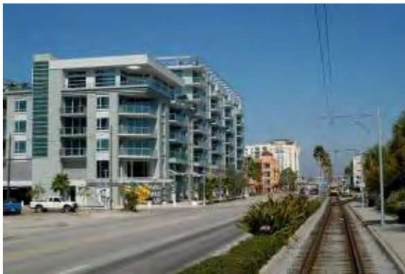
New residential development along the streetcar line near the harbor.
