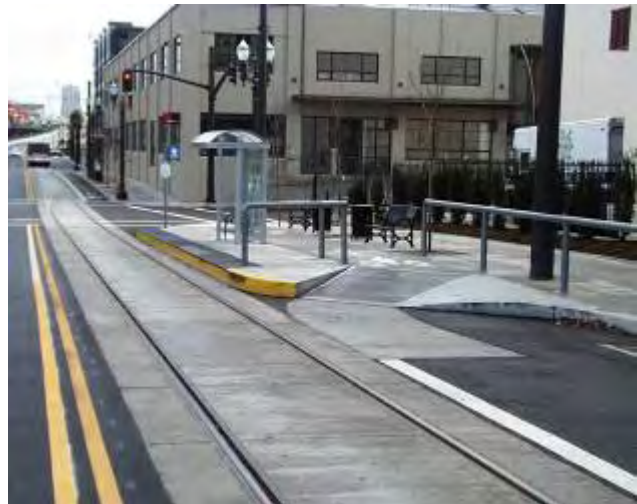
A slight raised platform extends from the curb to the rails at a streetcar stop.
