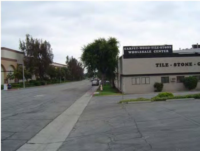
Figure 4.1-1: M&O Facility in Monrovia Site - View 1 1
