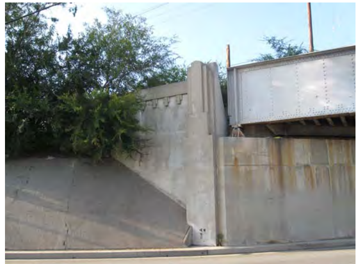
Figure 4.1-8: N. Colorado Boulevard Bridge Replacement View 2 8
