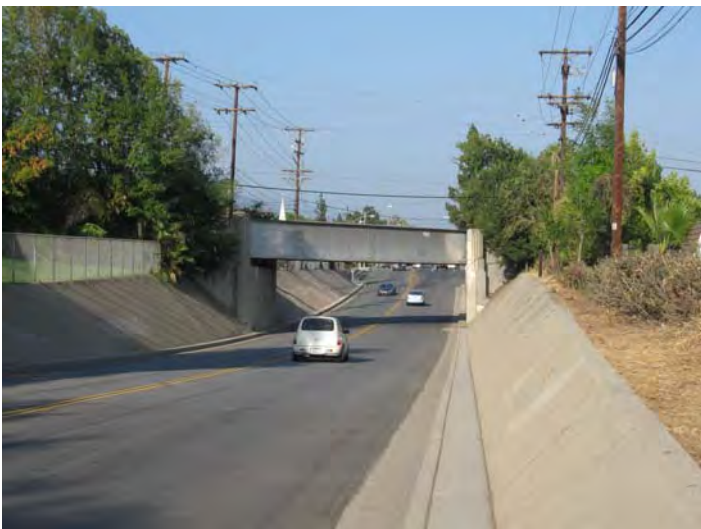
Figure 4.1-7: N. Colorado Boulevard Bridge Replacement View 1 7
