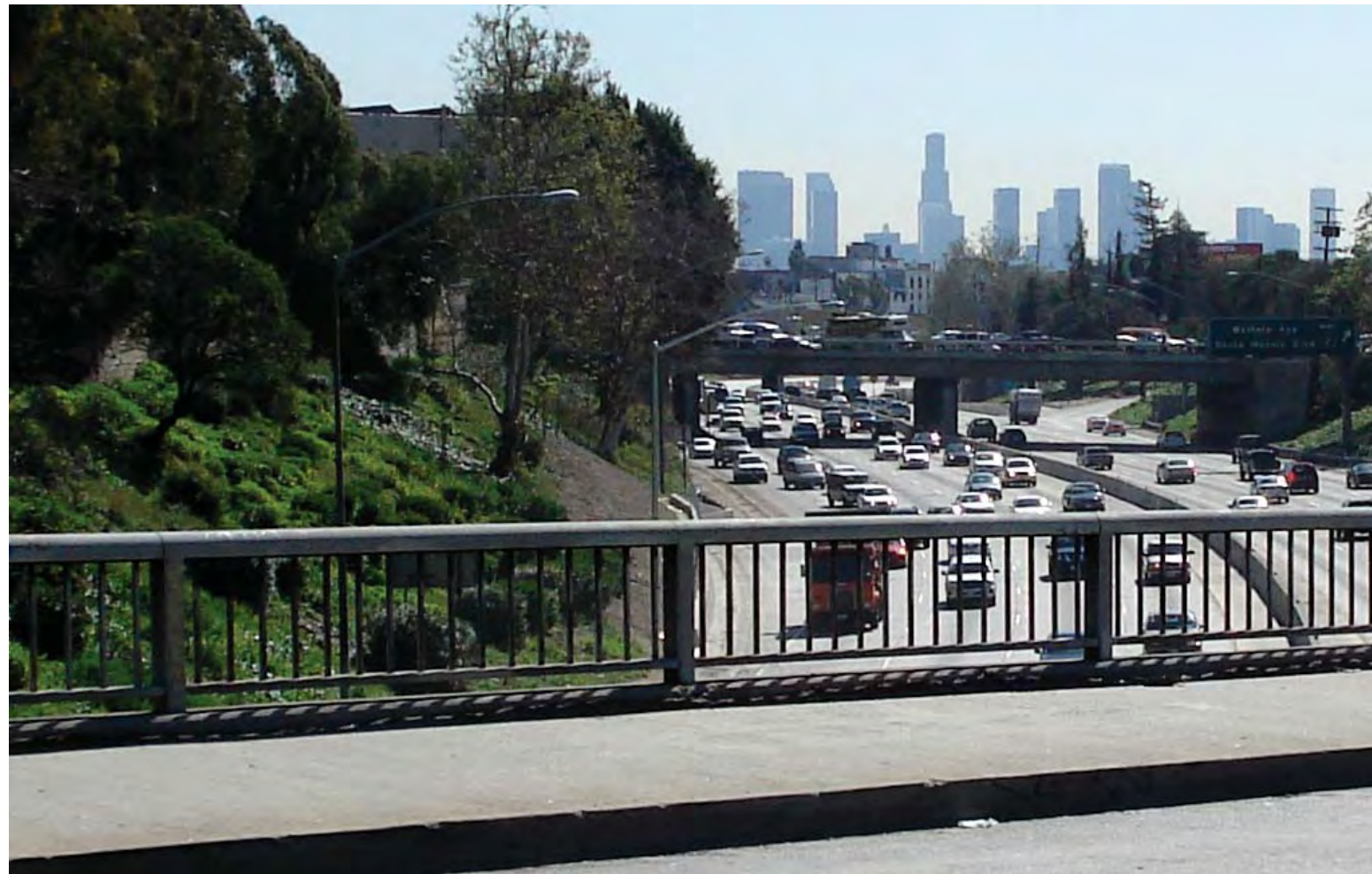
Existing ~ Fountain Avenue overpass and freeway, Western Avenue and downtown skyline in the distance
