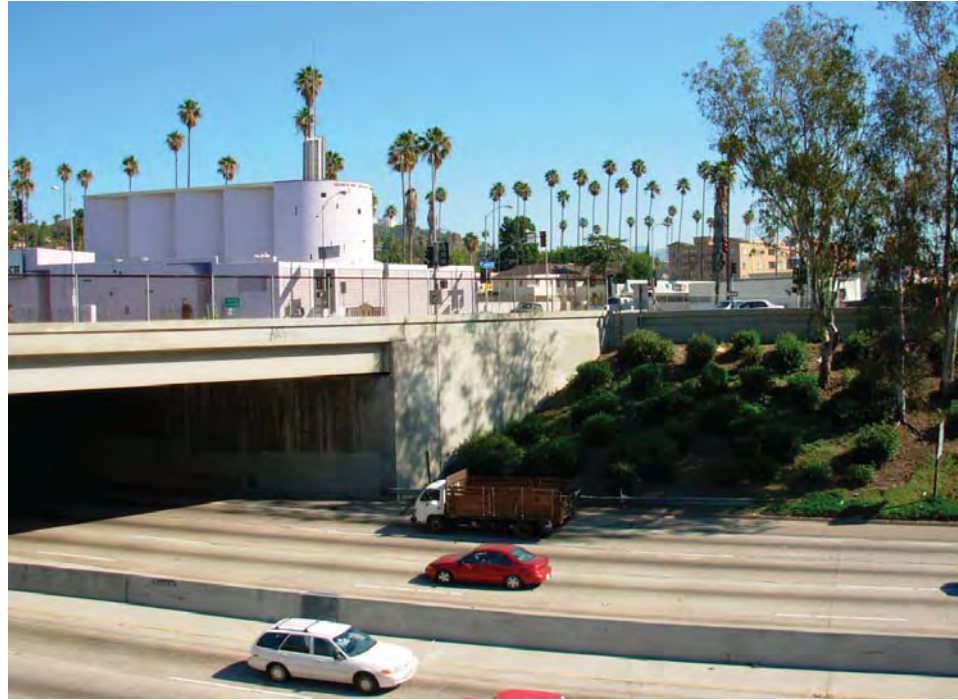
Hollywood Boulevard freeway overpass
