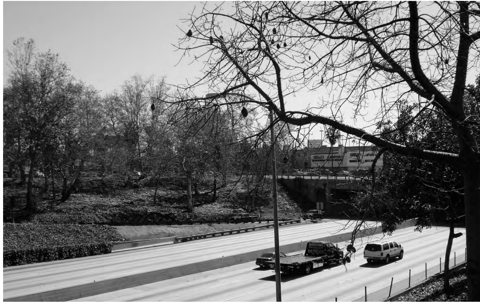
Existing ~ Sunset Boulevard off-ramp, overpass and freeway
