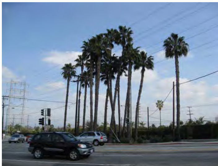
Cluster of Palm and high tension power poles at Fairfax Ave and La Cienega Blvd.
