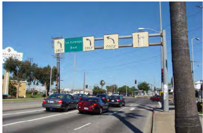
Three eastbound left turn lanes at La Cienega Boulevard and La Tijera Boulevard.
