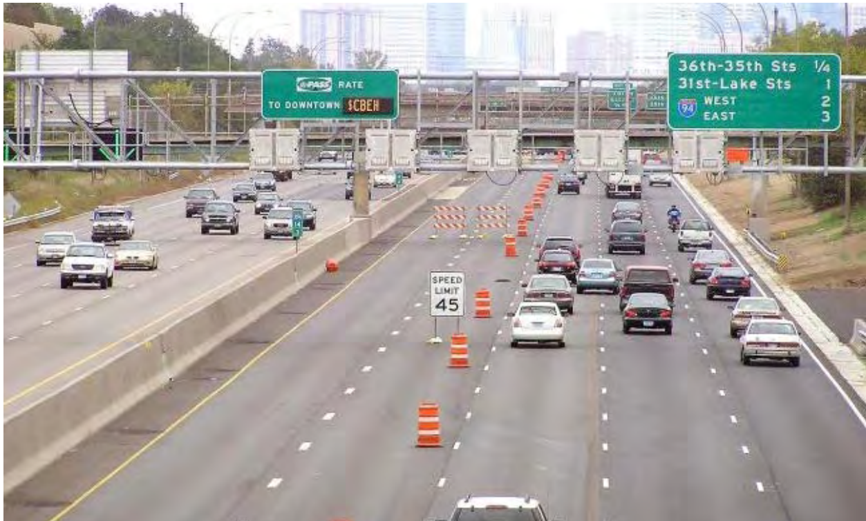
The MnPASS or congestion pricing lane on the left will be available at no cost to buses, car pools and to single driver vehicles willing to pay as little as 25 cents or up to $8 a trip depending on traffic levels. Traffic managers adjust the price in order to keep the lane flowing at 50 miles per hour. Photo by Dan Olson, Minnesota Public Radio
