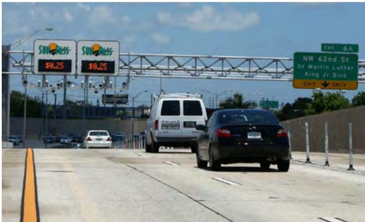
Express lanes using the SunPass technology in Florida. Photo courtesy of the Florida Department of Transportation.
