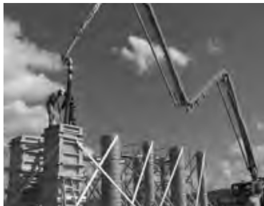
Half-scale reinforced concrete bridge columns for Phase II testing described in NCHRP Report 645 are cast with a concrete pump truck and consolidated with a hand vibrator at the Southwest Research Institute test site in Yancey, Texas.
