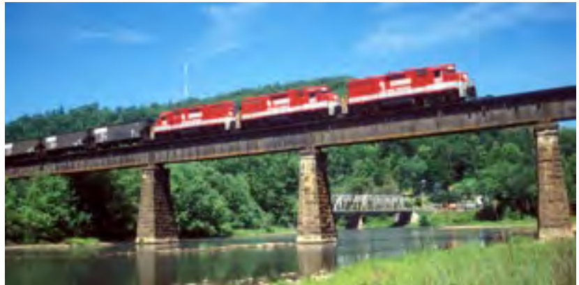
In early 2010, R. J. Corman Railroad Group received a Transportation Investment Generating Economic Recovery (TIGER) grant of $17.5 million for its Appalachian Regional Shortline Project rehabilitating railroads in Kentucky, Tennessee, and West Virginia. The Transportation Law Committee examined the legal implications of increased spending on railroads and other legal issues in transportation this year. (Photo: R. J. Corman Railroad Group)
