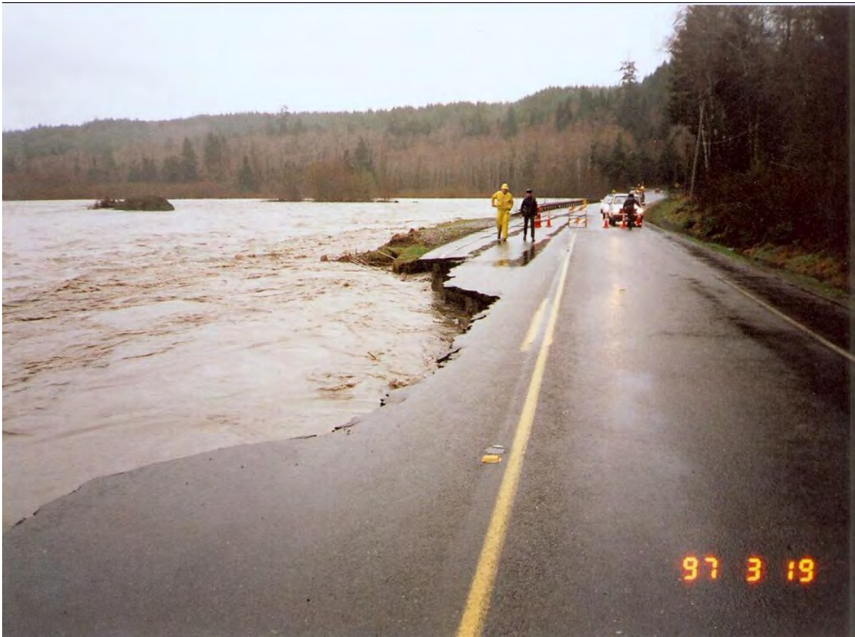
Changes in river dynamics: Hoh River flooding, channel migration, and avulsion. (Photo courtesy of Washington State DOT.)
