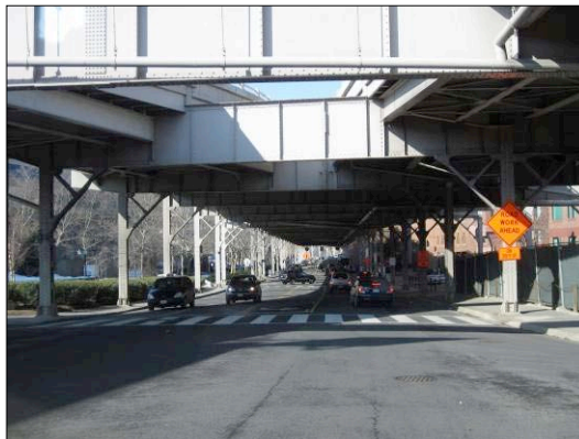
Figure 14: The Whitehurst Freeway looms above K Street
