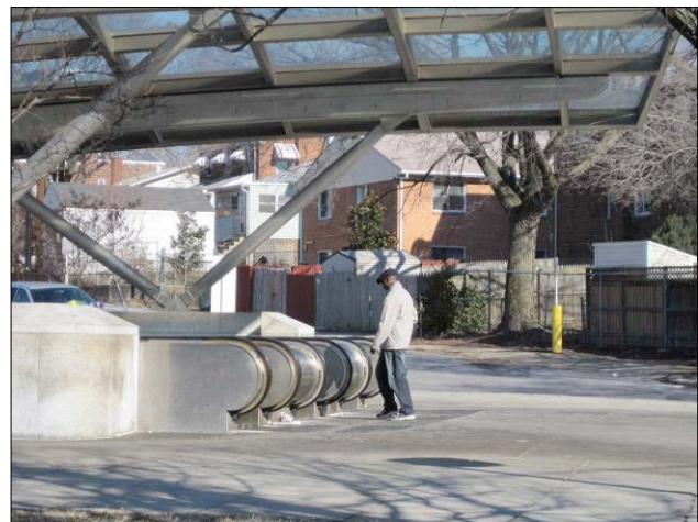
Figure 12: Benning Road Metro Station Entrance
