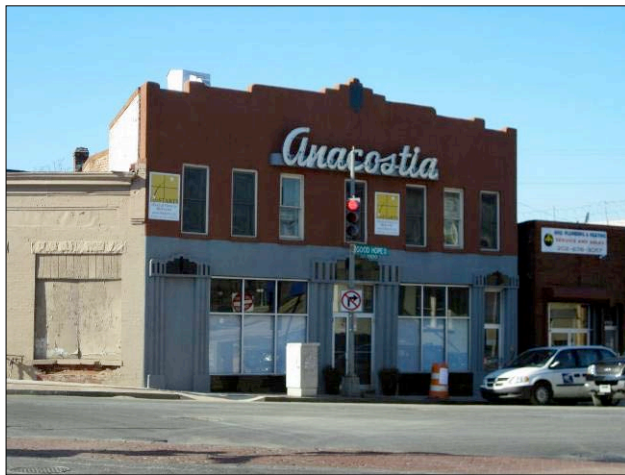
Figure 15: MLK Avenue at Good Hope Road
