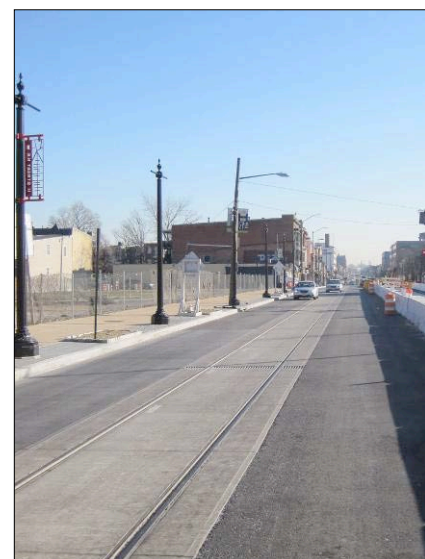
Figure 10: Recently installed rails at H and 2nd Street NE
