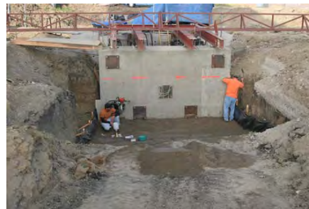
Placing Backfill for Abutment Test
