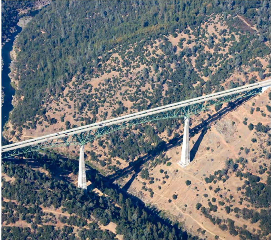
Figure 2-1. The Foresthill Bridge, spanning the American River in Placer County near Auburn, is to be retrofitted as part of the Local Seismic Safety Retrofit Program.
