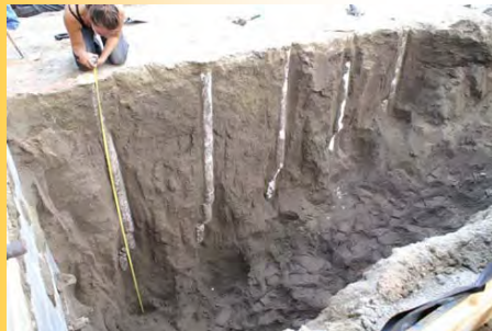
Excavation after Abutment Back-wall Test
