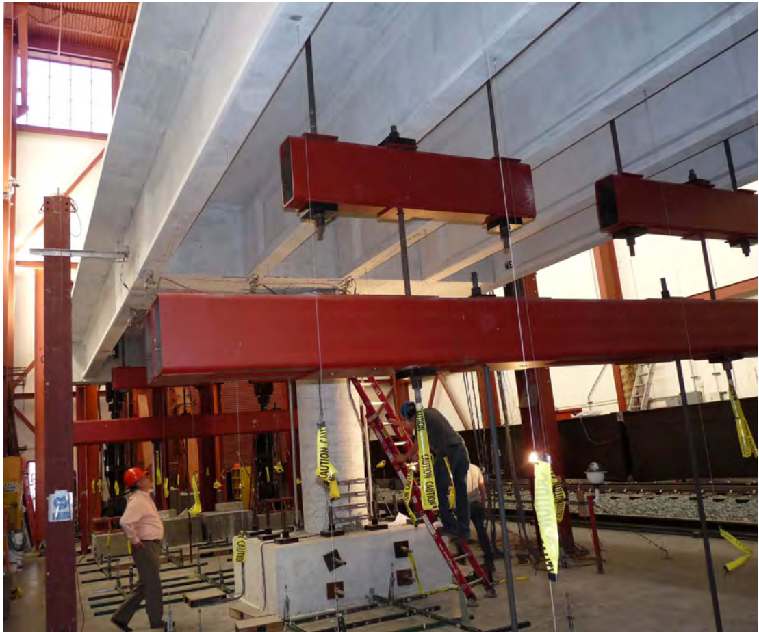
Figure 6-1. Results from large scale testing of precast girder system seismic performance will be used to update Caltrans seismic design criteria.
