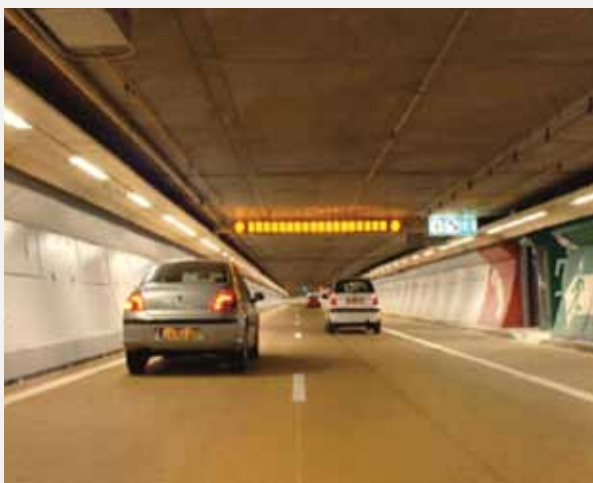
The first toll tunnel has two low-clearance decks and is exclusively for light-duty vehicles. The second tunnel is of traditional style.
