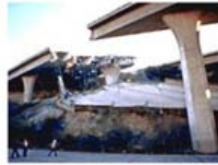
Highway vulnerability to Northridge Earthquake
