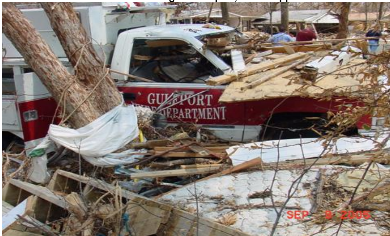
FIGURE 1: Hurricane Katrina Damage in Gulfport, Mississippi.
