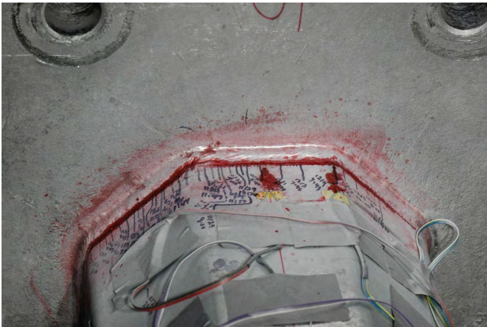
Figure 53 Fatigue cracking in arm of specimen VII-5, from the fillet weld toe on the tube in tube-to-transverse plate connection
