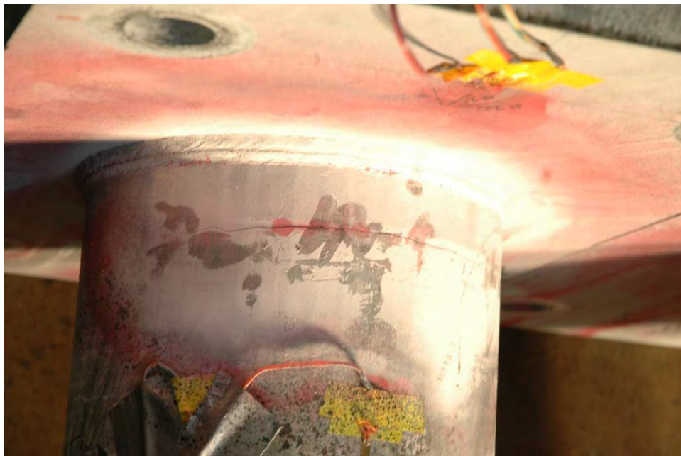
Figure 42 Fatigue cracking in arm from the toe of backing ring to tube weld (inside)
