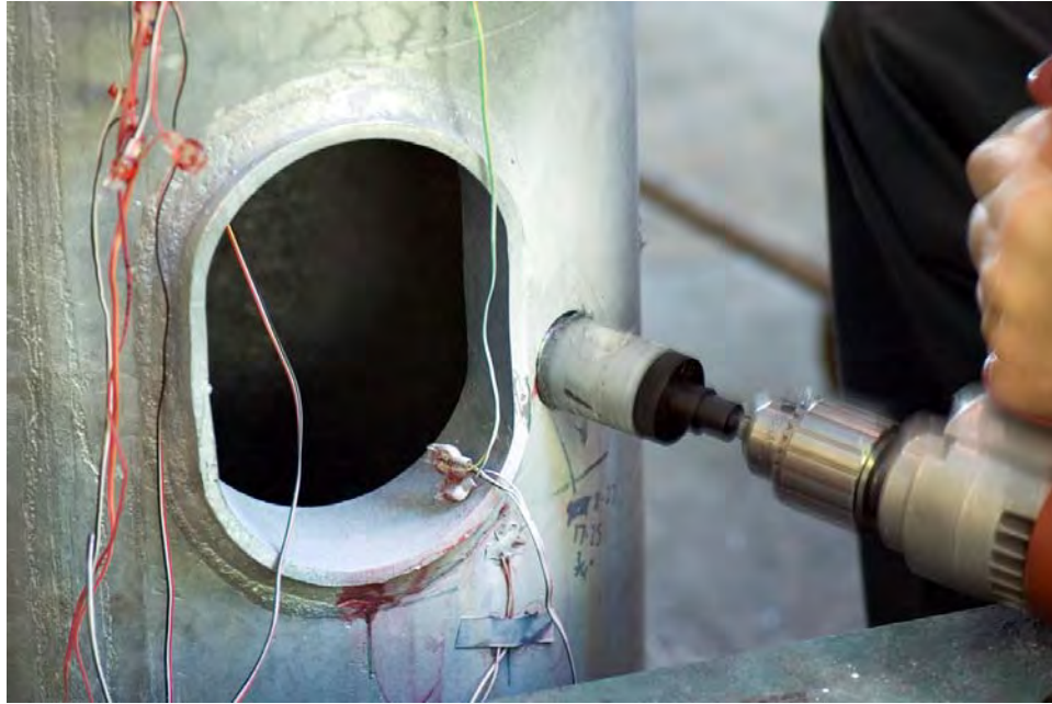
Figure 41 Holes drilled at the crack tip for continuing fatigue tests
