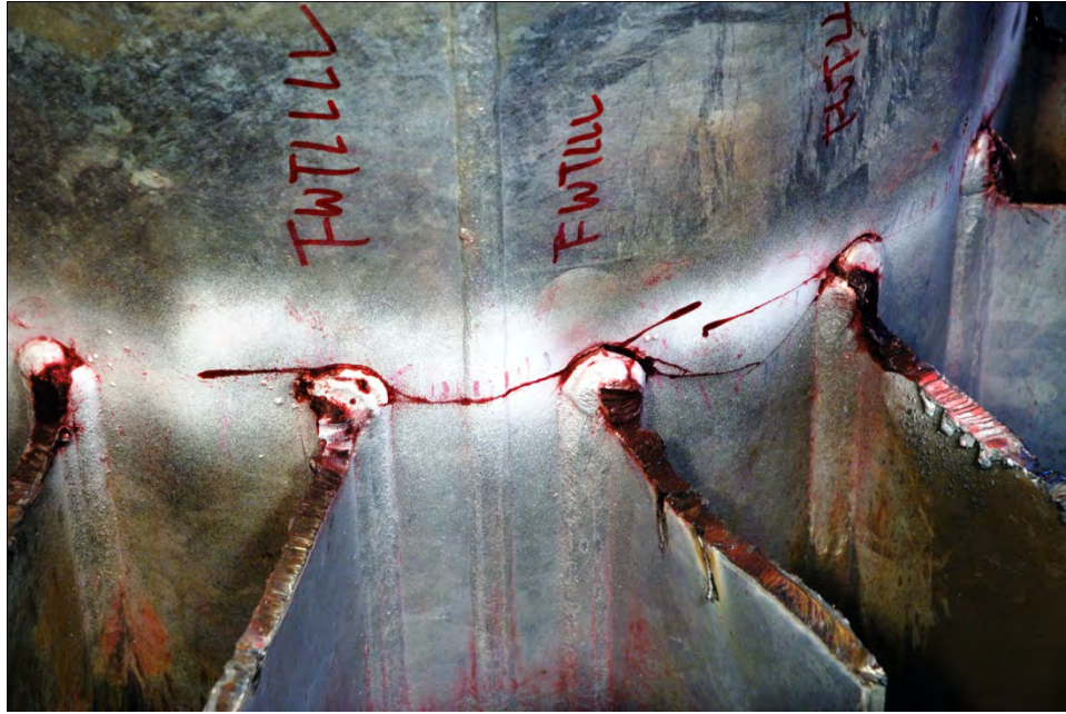
Figure 56 Fatigue cracking in specimen IX-3 from the stool stiffener to tube weld toe at the termination of the vertical stiffener on the tube wall (with stool top plate removed)
