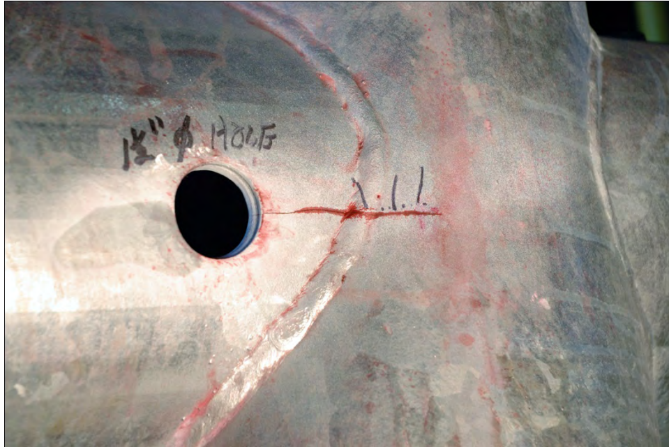
Figure 50 Fatigue cracking in specimen VI-1 from weld root arrested by hole drilling in the arm sleeve
