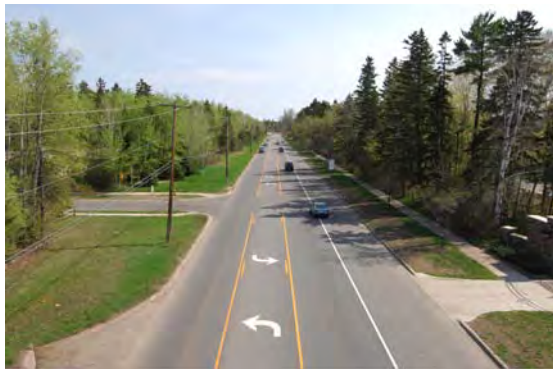
Existing London Road and 36 th Avenue, looking northeast
