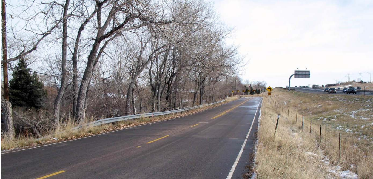
Figure 2. CDOT Test Site before Construction (Looking East)
