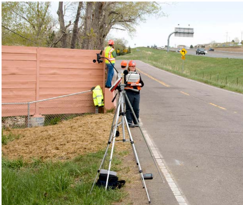
Figure 4. Measurement of Barrier Noise Reduction (Looking East)
