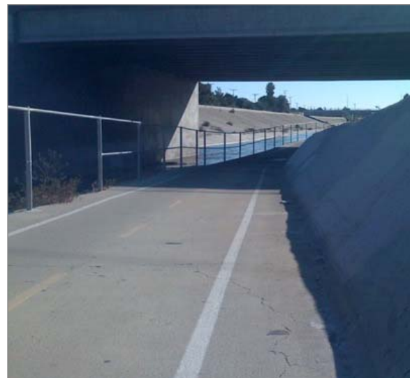
Undercrossings provide key connections and allow path users to avoid a potentially dangerous at-grade crossing of a major street.
