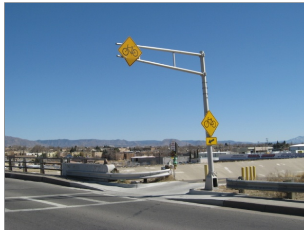
Type 1 crossings include signage and pavement markings.
