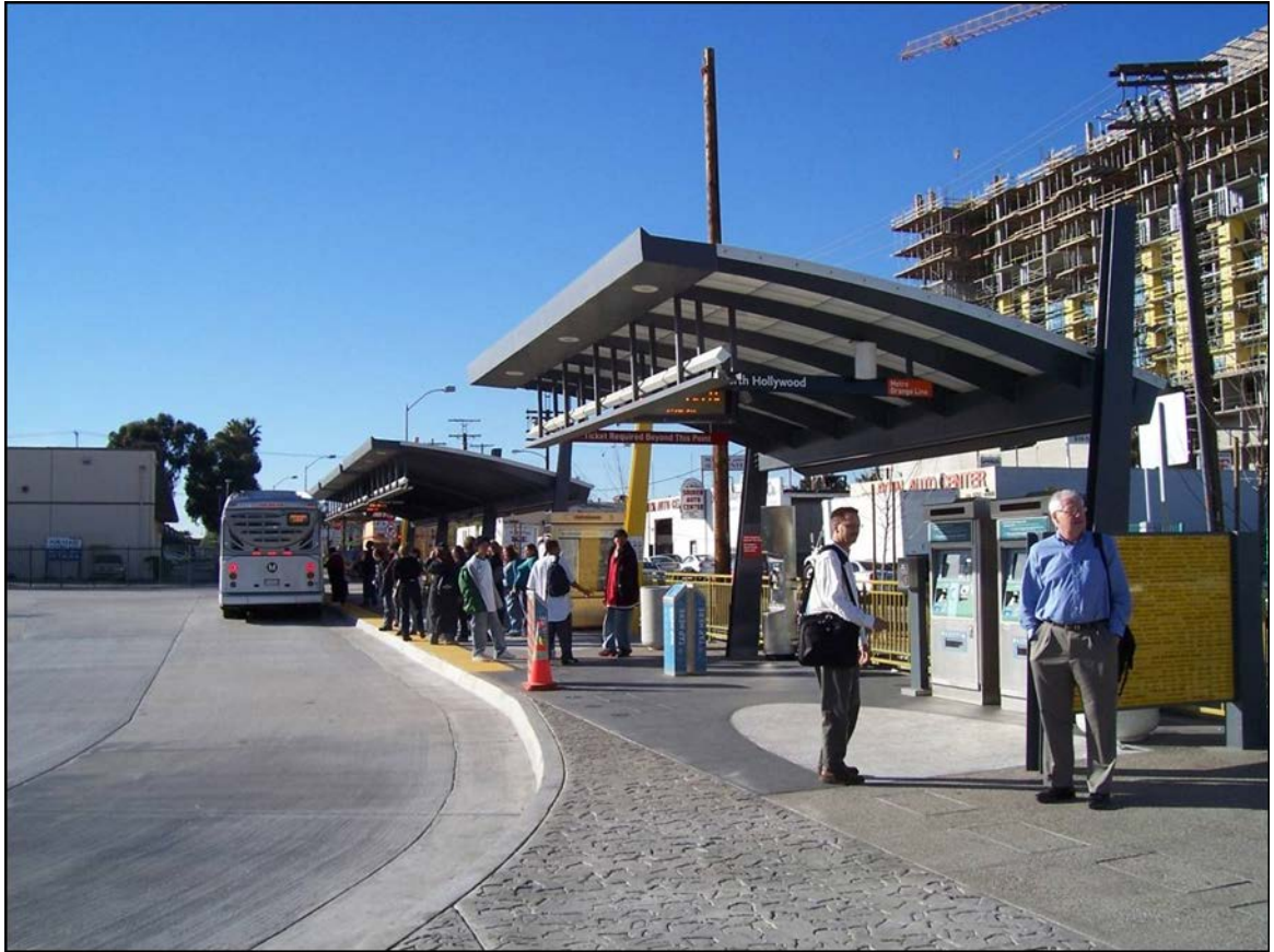
Figure 5-4 Construction at Orange Line Terminus and Red Line Connection at North Hollywood Station
