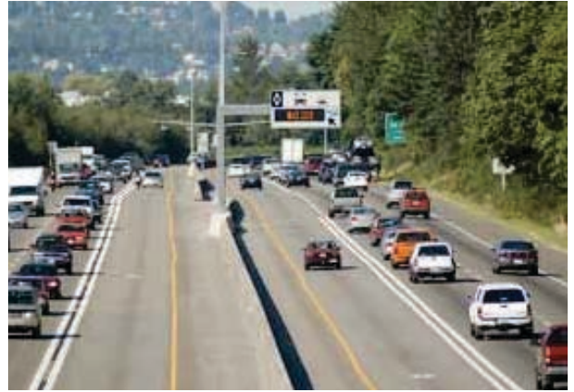
HOT lane user rates are displayed on digital boards above a free-flowing HOT lane in Washington State.
