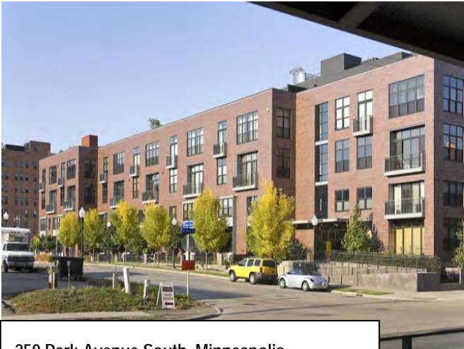
250 Park Avenue South, Minneapolis Adaptive Reuse Condominium project Near Downtown East/Metrodome Station Source: minneapolisloftsandcondos.com
