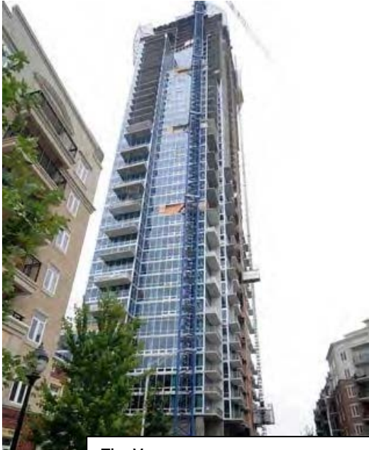
The Vue 50-Story condominium project, Uptown Charlotte (under construction). Source: Charlotte Observer
