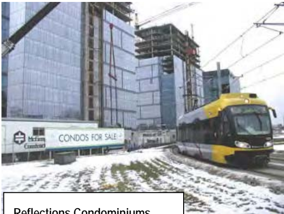
Reflections Condominiums (when under construction) High-rise condominium project near Bloomington Central Station Source: Metropolitan Council
