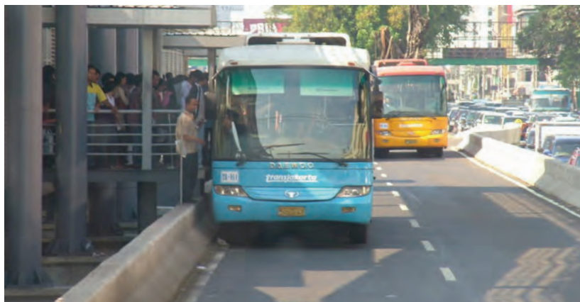
This Transjakarta line (Jakarta, Indonesia) includes a physically-separated passing lane at the station stop. Photo: ITDP
