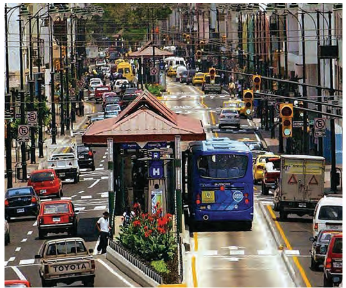
A dedicated one-directional BRT lane in the middle of a one-way street in Guayaquil, Ecuador. Photo: ITDP
