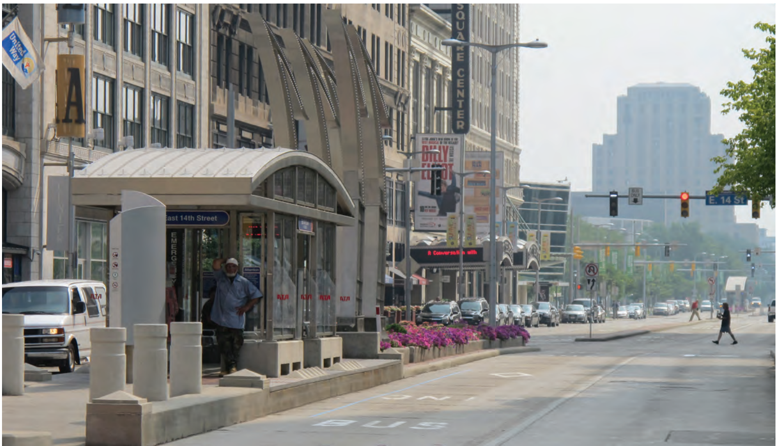
BRT station in Cleveland, Ohio, appropriately set back from the intersection. Photo: ITDP
