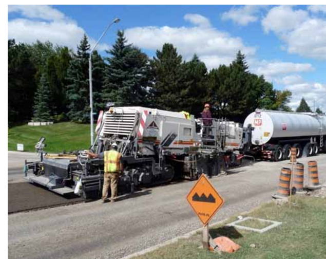
NCHRP Synthesis 421 gathers information on hot and cold in-place recycling and full-depth asphalt reclamation—processes that allow transportation agencies to reduce unnecessary traffic congestion during construction and optimize in-place materials.
