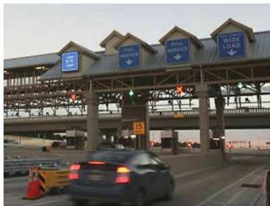
NCHRP Report 689 examines the direct costs of alternative systems of generating revenue, such as this electronic toll collection plaza in Austin, Texas. (Photo: Central Texas Regional Mobility Authority)
