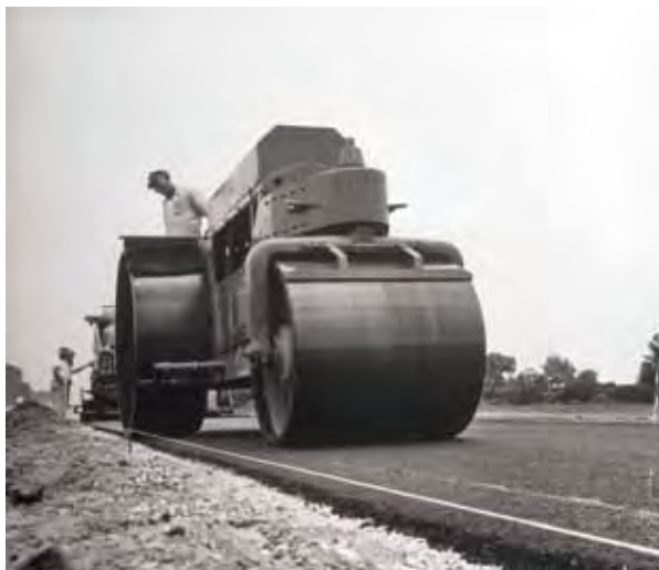
Construction of the New Jersey Turnpike in the 1950s.
