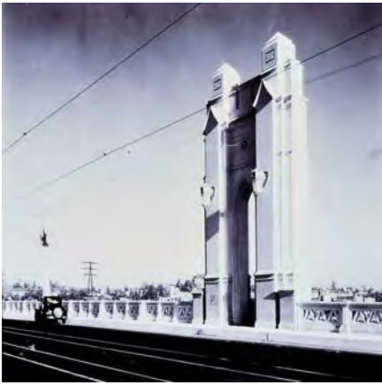
4 th Street bridge over the Los Angeles River
