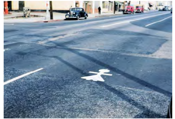
Unique pedestrian pavement marking
