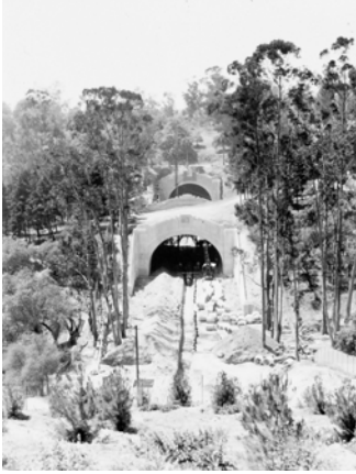
Construction of the Figueroa Street tunnels
