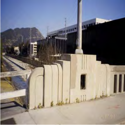
Lankershim Boulevard bridge over the Los Angeles River
