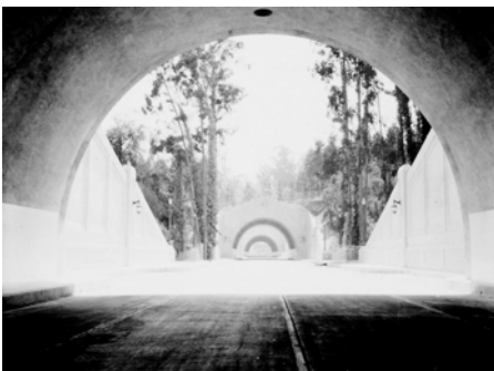
The original three Figueroa Street tunnels in 1931.
