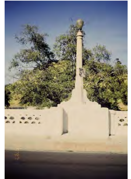
Avenue 60 bridge over the Los Angeles River
