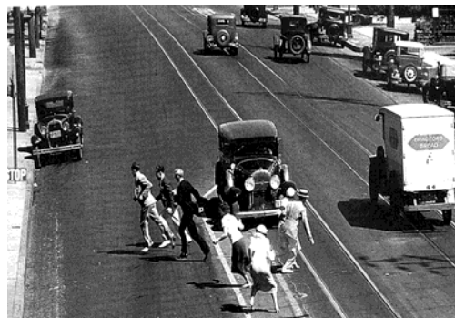
Staged safety photo
