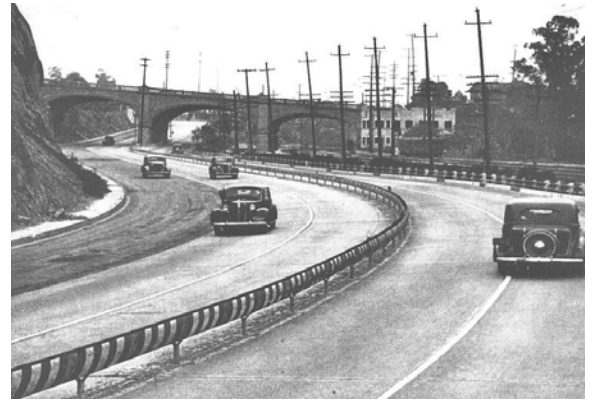
Ramona Parkway at the Macy Street Overcrossing, showing the special guard rail Graphic - 8090
