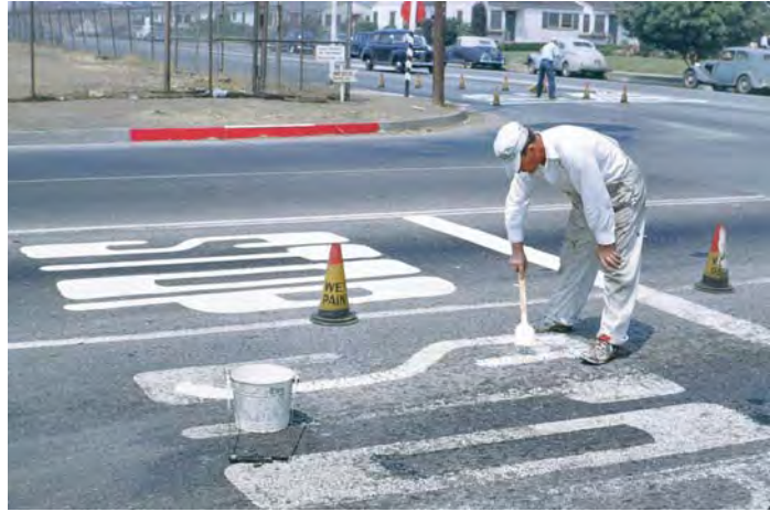
Pavement message maintenance using a brush, circa 1950
