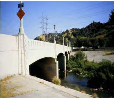
Riverside Drive bridge over the Los Angeles River near Griffith Park
