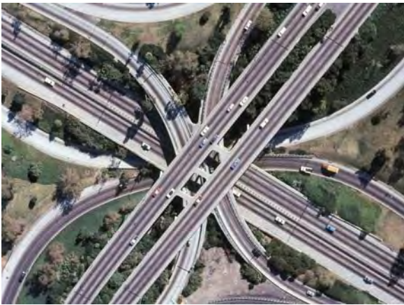
The Four Level Interchange, the first full-freeway interchange, circa 1951 Graphic - 3020
