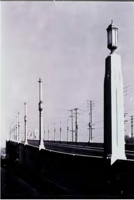
6 th Street bridge over the Los Angeles River
