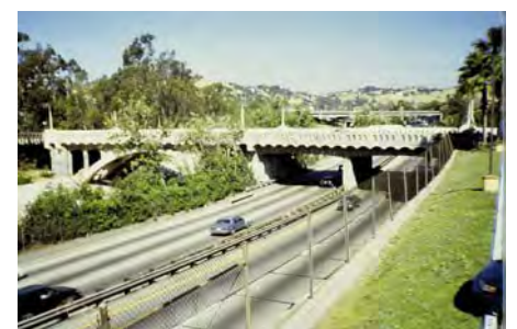
Avenue 26 bridge over the Arroyo Seco
