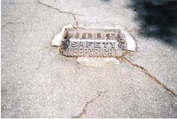
Metal pavement marking from the 1920's
