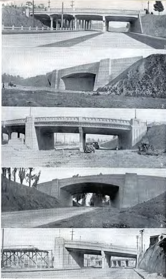
GRADE CROSSINGS ARE ELIMINATED on the new Ramona Boulevard by seven bridges, five of which are shown above. No. 1—Eastern Avenue, a reinforced, concrete girder structure which the State extended with a 39-foot, 6-inch span providing a 60-foot roadway and 2-foot 8-inch sidewalks. No. 2—Coyote Pass grade separation, a 140-foot concrete girder structure providing a 60-foot roadway and 2-foot, 4-inch sidewalks. No. 3—State Street, a concrete girder structure extended by the State with two 44-foot spans providing a 40-foot roadway and two, 2-foot, 5-inch sidewalks. 4—Monterey Pass, an 87-foot concrete girder span providing a 60-foot roadway and two 4-foot sidewalks. This structure permits Monterey Pass traffic to pass under Ramona Boulevard. No. 5—Marengo Street, a 112-foot reinforced concrete girder extension of the existing bridge. Provision is made in the next biennial budget for extending the concrete construction to replace the old section of bridge.
