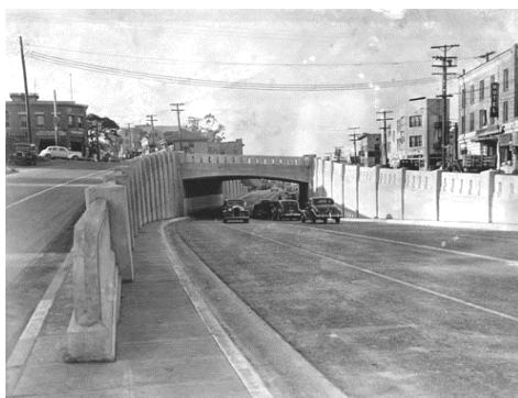
Construction of the Figueroa Street grade separation and diamond interchange at Temple Street.
