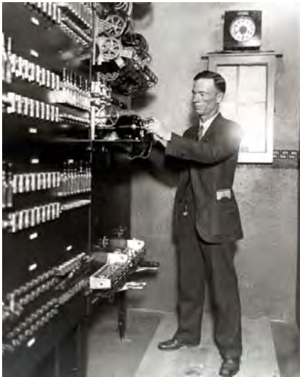
Acme Signal Center in Pershing Square basement, circa 1924 Graphic - 3080
