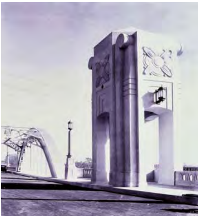
6 th Street bridge over the Los Angeles River
