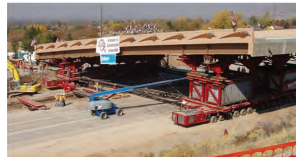
Moving the superstructure using SPMTs.
