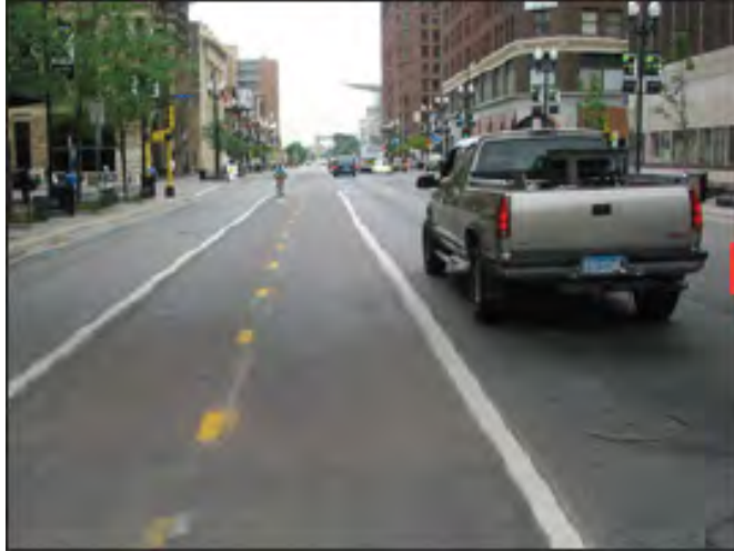
Figure 3.8 - Hennepin Avenue prior to lane reconfiguration in 2009
