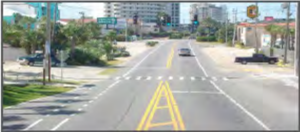
Figure 1.5 - Photograph taken on Front Beach Road
