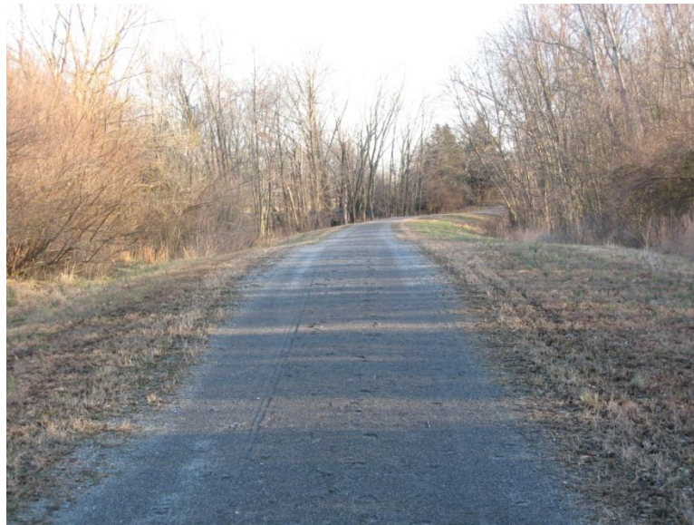
Figure D.17. Road bed offers support across trail width.
