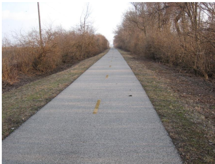
Figure D.38. Good edge support and vegetation clearance.
