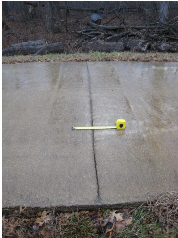
Figure D.26. Typical tooled contraction joint.
