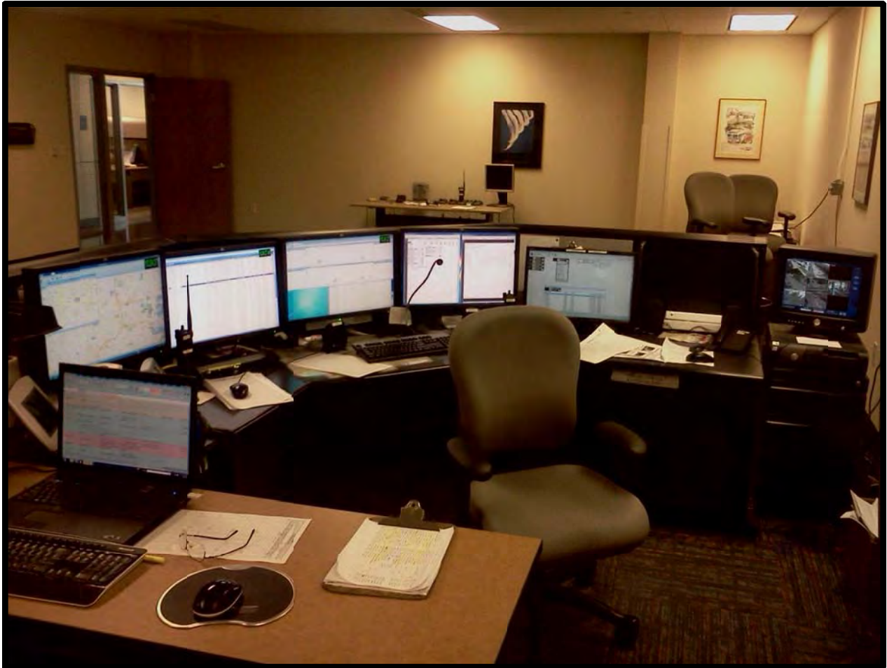
Figure 3-2 Radio Control Room – South County Station
