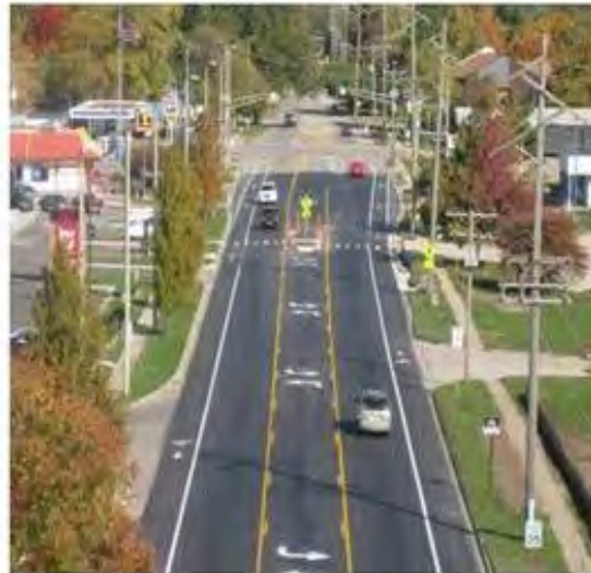
Complete street with center turn lane, bike lane and pedestrian refuge island at bus stop.
