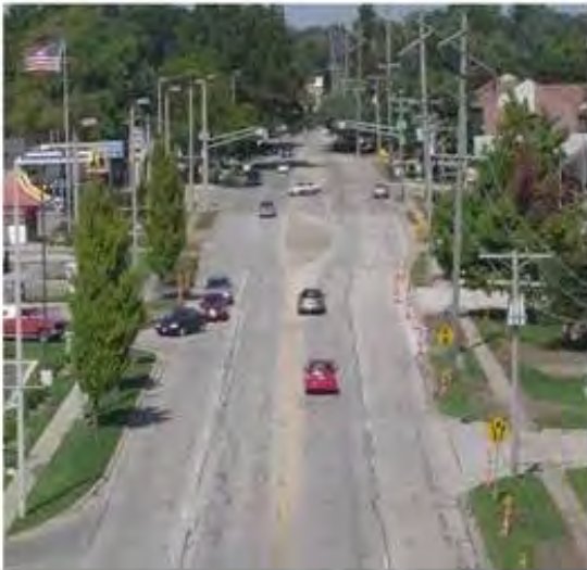
Original four-lane arterial designed to maximize motor vehicle traffic speeds.
