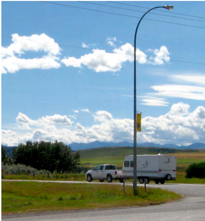
Rural intersection lighting.
