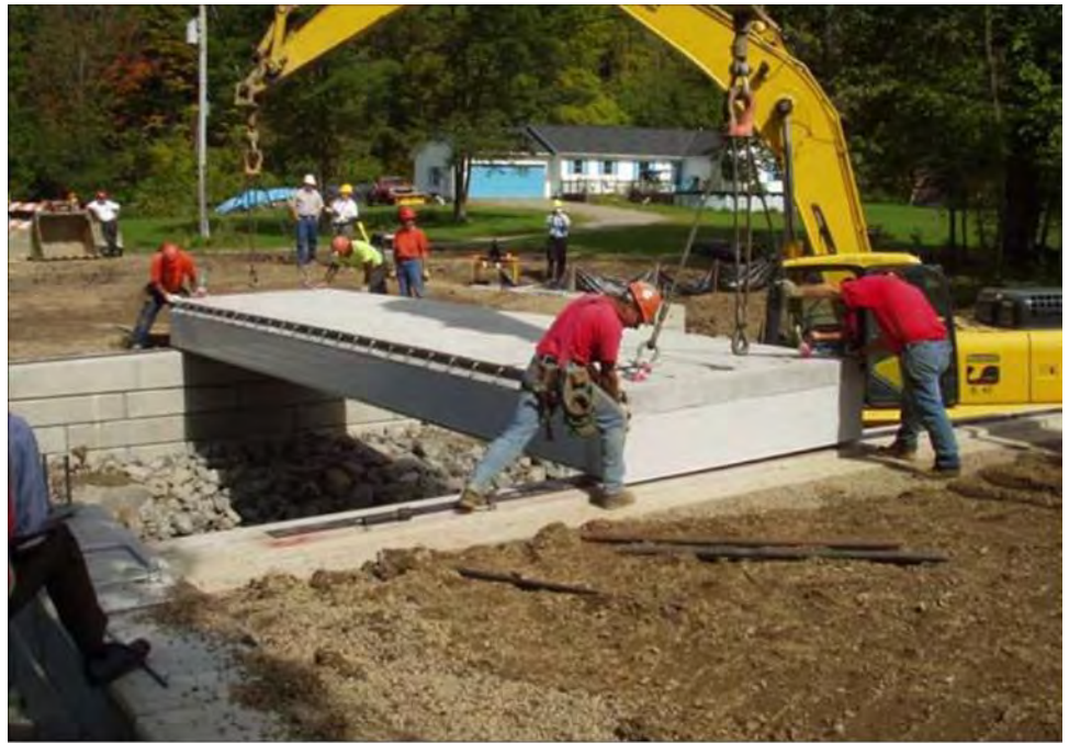
Figure 3: Prefabricated Bridge Elements at Construction Site
