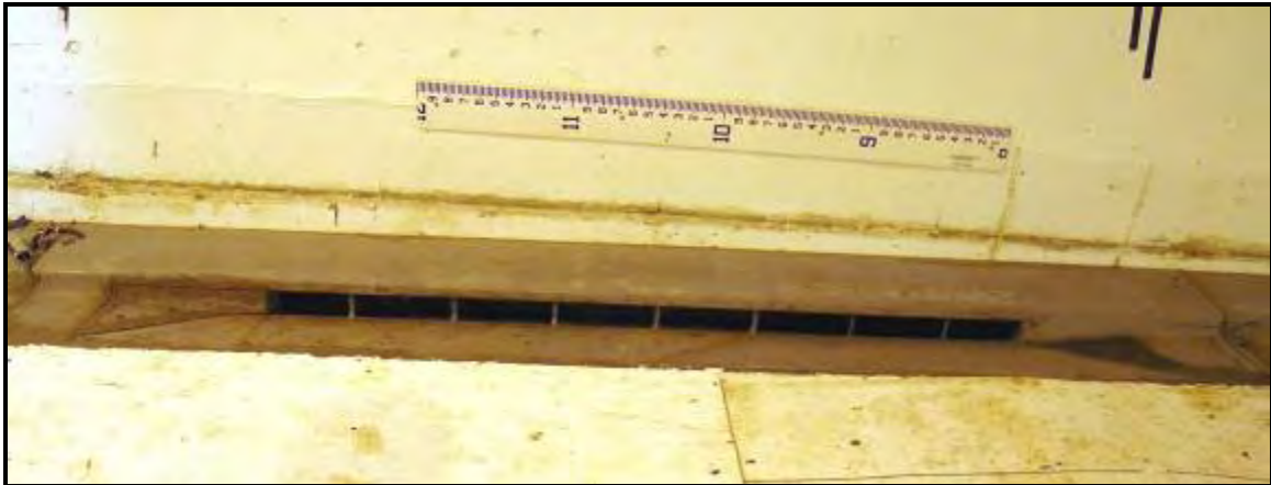
Figure 3.25 R15 Curb Inlet Photograph
