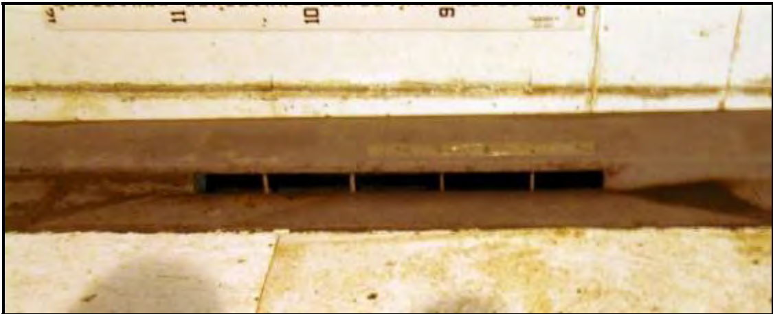
Figure 3.23 R9 Curb Inlet Photograph
