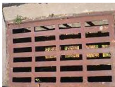
(a) grate inlet
