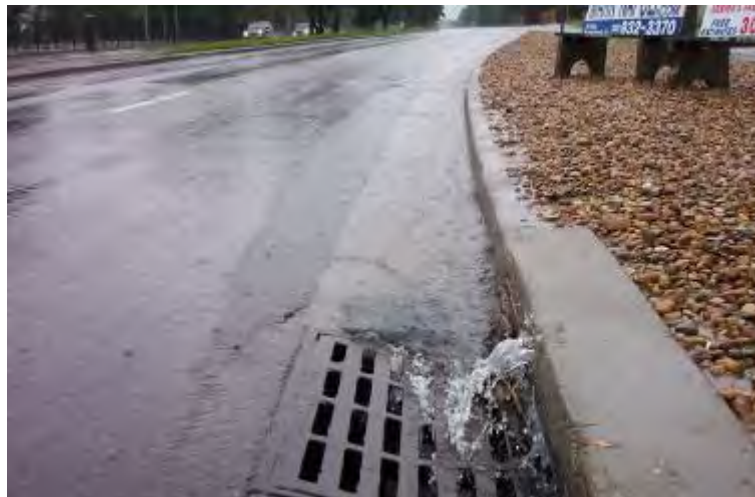
Figure 7.1 Splash-Over Flow Over Type 13 Grate
