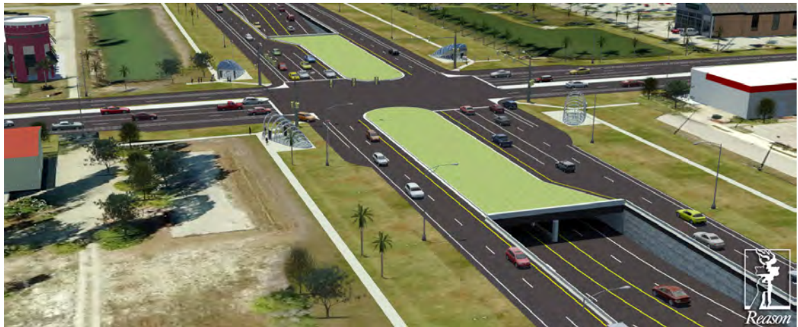
Figure 5: Typical Arterial Underpass
