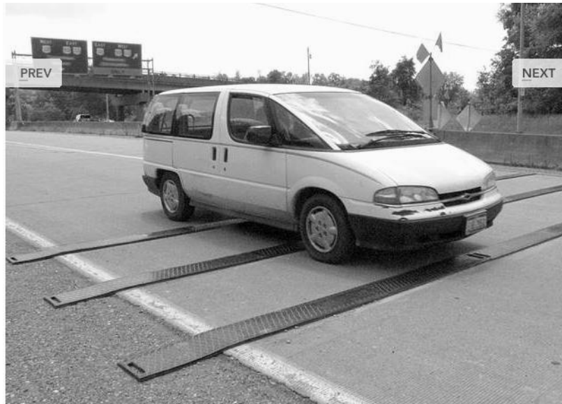
Figure C.1. Temporary rumble strips
