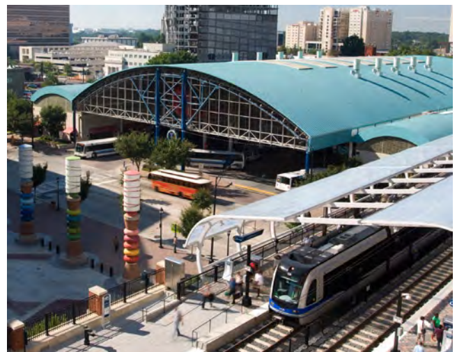
Charlotte, North Carolina has used New Starts grants for their Blue Line light rail — including an upcoming expansion that received funding in October 2012.
