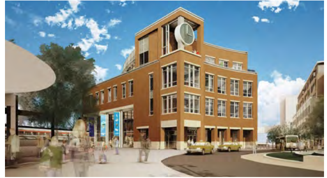
Normal, Illinois, used Bus Facility Grants to build their new multimodal center that also includes Amtrak service.
