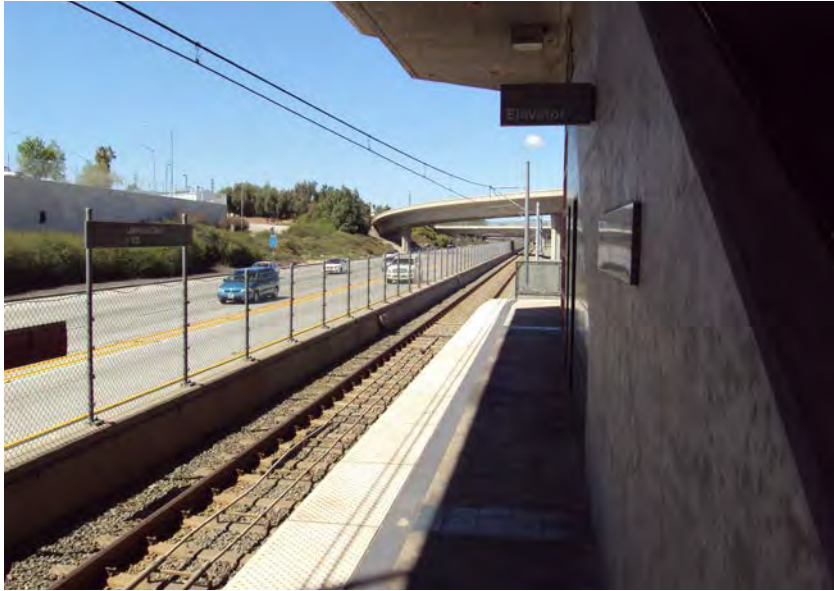
Figure 5: Wall Formed by Stairway at Lakewood Station
