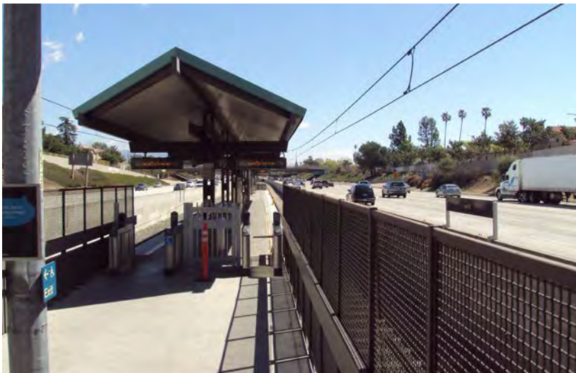
Figure 6: View of Canopy at Lake Station
