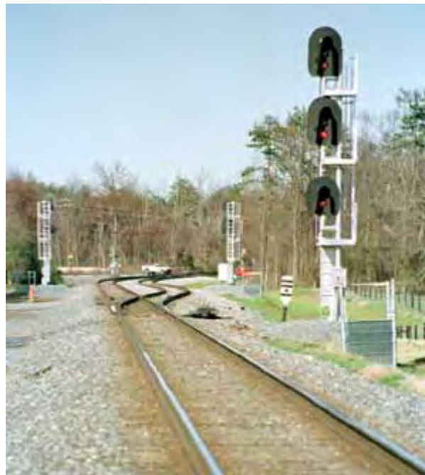
Figure 11: Control Point with Three Signal Heads
