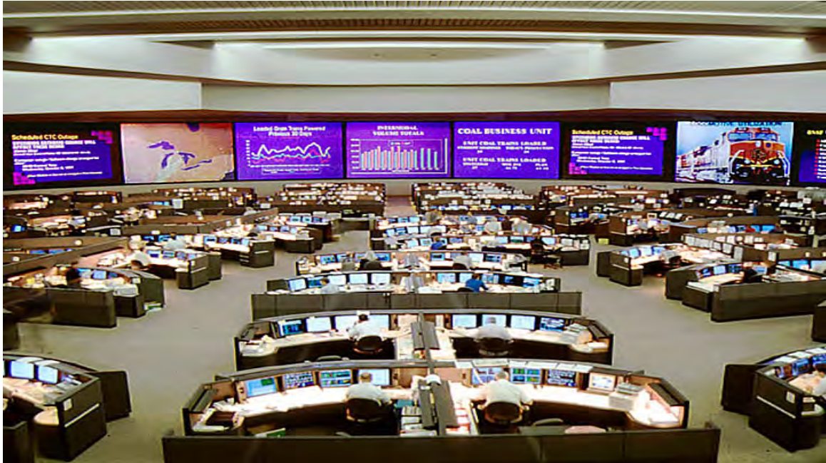
Figure 4: BNSF Network Operations Dispatch Center
