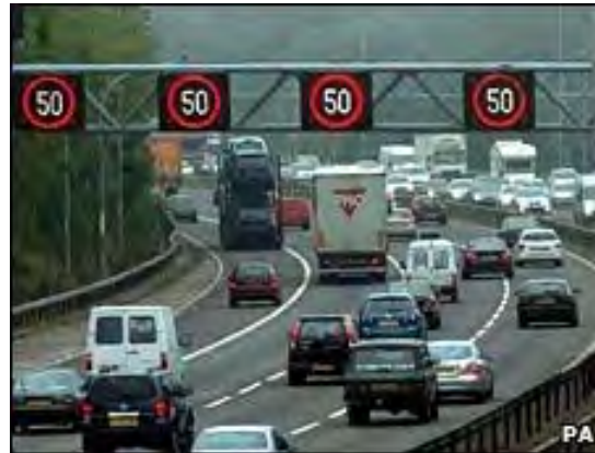
Figure B-3. VSL Sign on M25 Motorway in the UK (Robinson 2000)
