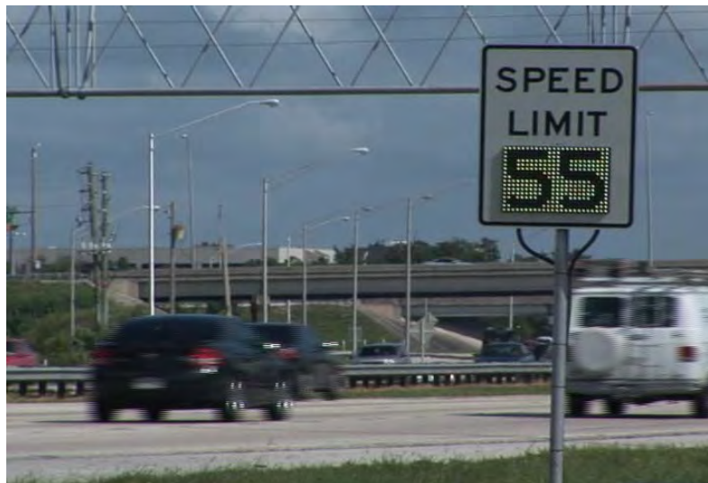
Figure B-4. Variable Speed Limit Sign on I-4 in Orlando, FL
