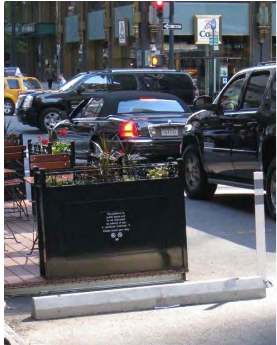
Figure 41. Flexible bollard and wheel stop, New York City, NY. Credit: NYC Department of Transportation
