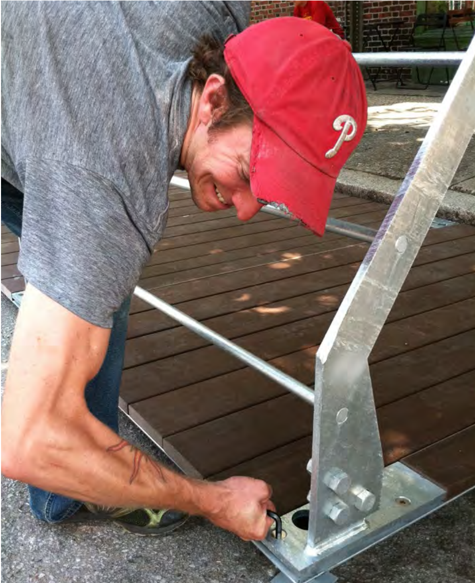
Figure 69. Parklet installation, Philadelphia, PA. Credit: Philly Bicycle Coalition
