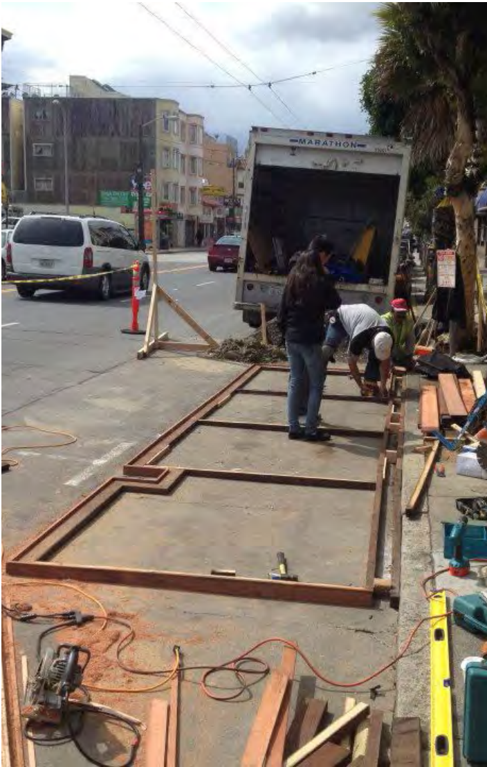
Figure 84. Wooden sub-structure, San Francisco, CA. Credit: Excelsior Action Group / www.eagsf.org
