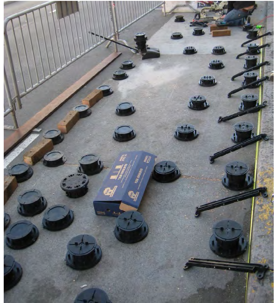
Figure 79. Bison pedestal system during installation, San Francisco, CA.
