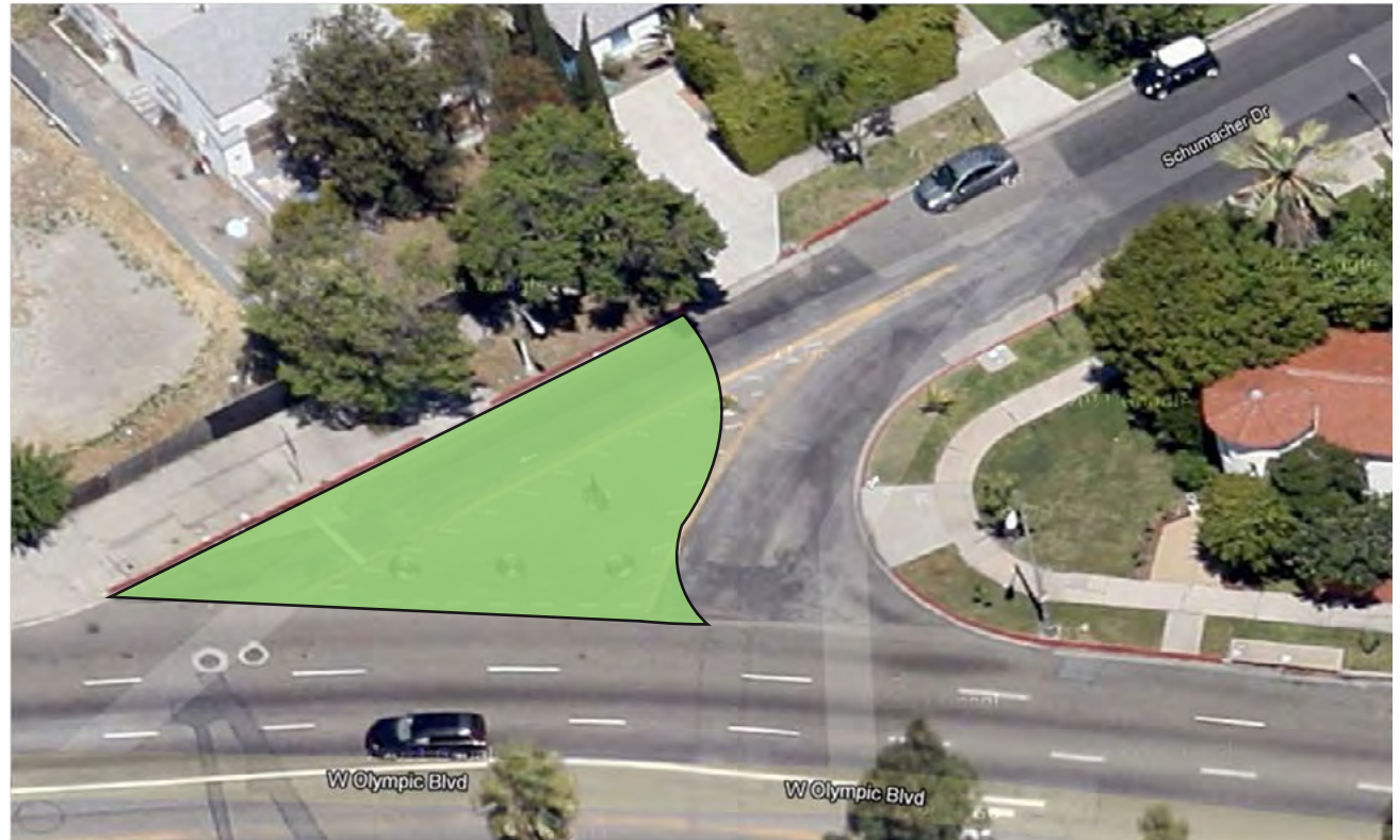
Figure 111. Concept for “residential parklet,” Los Angeles, CA. Credit: India Brookover/ Google Maps
