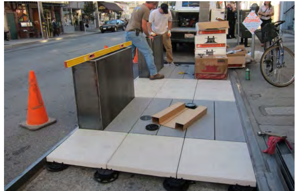
Figure 81. Pre-cast concrete pavers during installation, San Francisco, CA. Credit: Streetsblog SF
