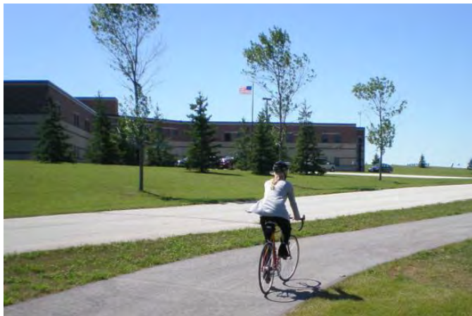
Figure 39: Students, Faculty, and Staff Use the Path to Walk and Bicycle to School (source: Sheboygan County NOMO)
