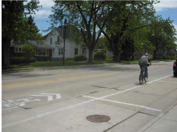
Figure 37: The New Sidewalks and Bicycle Lanes along South Main Street Provide Safe Spaces for Bicycling and Walking (source: Sheboygan County NOMO)
