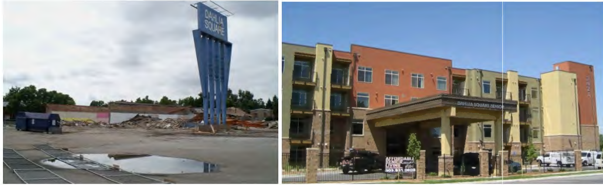
Figure 3. A deteriorating and underused shopping center (left) in Denver, Colorado, was redeveloped into Dahlia Square Senior Apartments (right), which provides affordable homes next to a new medical center. Photo credit: EPA.
