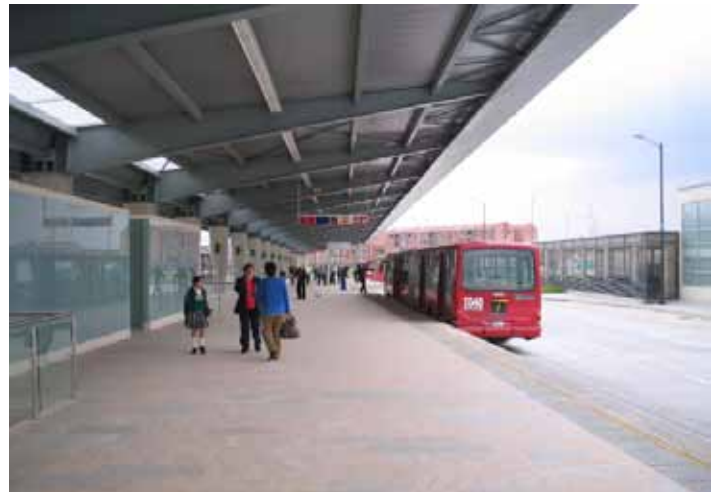
Images showing a typical layout for a TransMilenio terminal. Above: the green feeder buses stop on the left side of the platform. Below: the articulated red trunk line buses stop on the right side of the same platform. EMBARQ photos.
