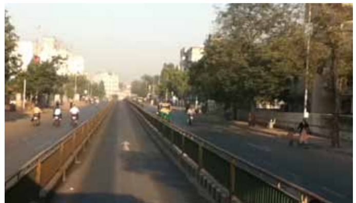
Guardrails between the bus lane and the mixed traffic lanes on the Janmarg BRT corridor in Ahmedabad. EMBARQ photo.
