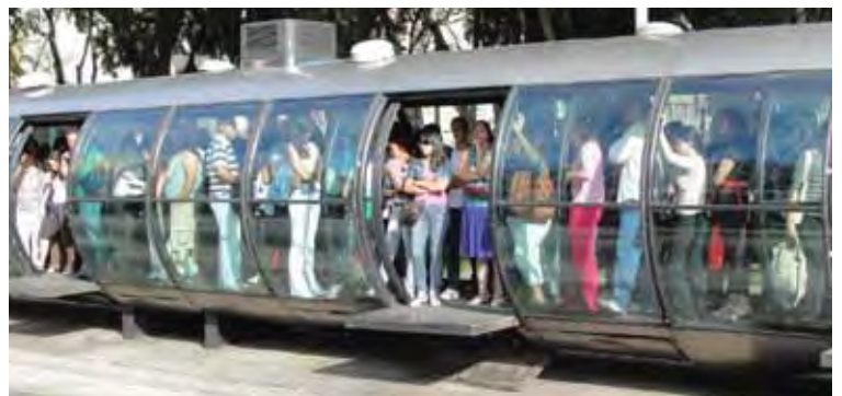
A platform screen on a BRT station in Curitiba. The doors are open, even though no bus is present. This is a safety risk in a crowded station, as passengers can accidentally fall in the bus lanes. Photo courtesy of EMBARQ Brasil.
