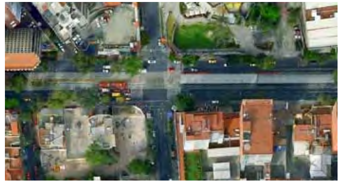
A narrow four-leg intersection along Metrobus Line 1 in Mexico City. Google Earth image.
