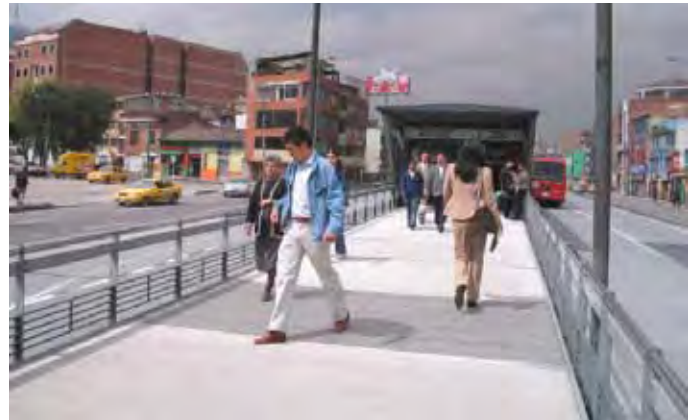
TransMilenio 2006: a pathway between two sub-stops at the same station. Note the low guardrails, approximately 1 meter in height. Because they were so low, people could jump over them easily, and this was a major pedestrian safety risk. EMBARQ photo.
