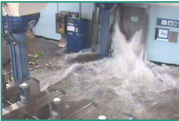
▲ Hoboken PATH Station Flooding. Photo Credit: ABC News
