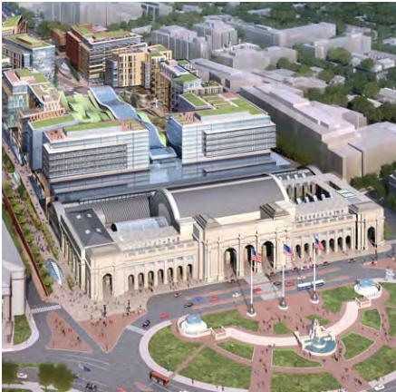
View of the historic station, train shed and air rights development from the southwest. Image courtesy of Akridge/SBA.
