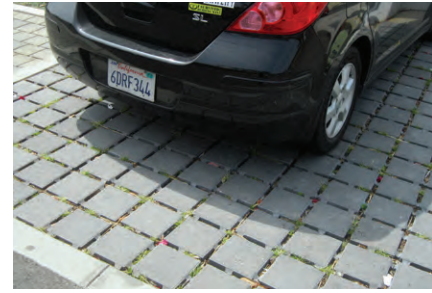
3 Stormwater is infiltrated through the use of permeable paving systems, landscape planters and other purposely located pervious surfaces.
