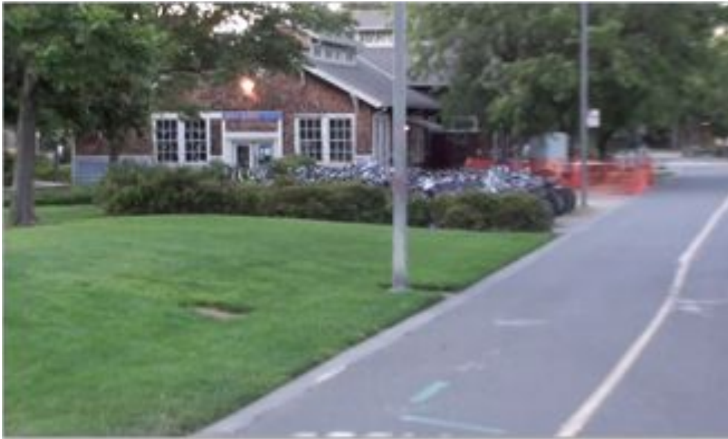
Figure 56. Repair Facility with Storage Lot at Bicycle Station – Davis, California
