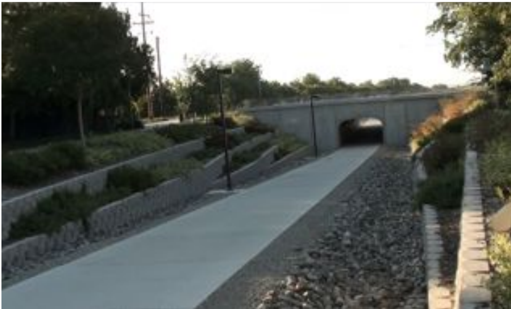
Figure 47. Underpass for Bicycle Path #2 – Davis, California
