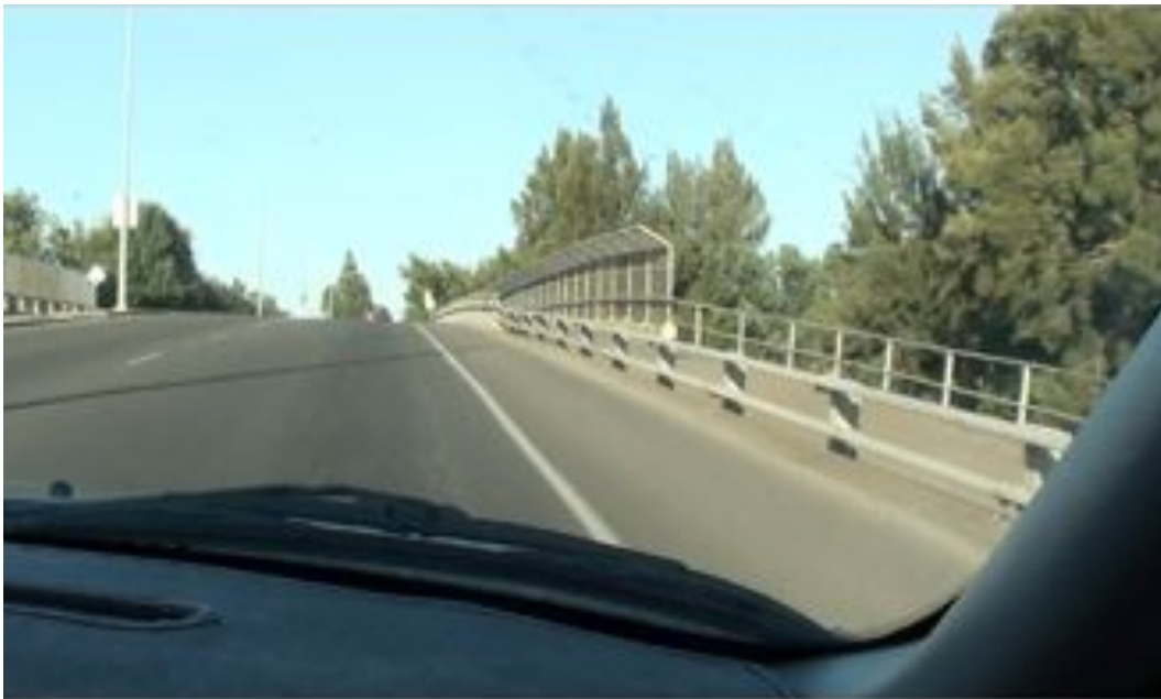
Figure 48. Bicycle Lane on Highway Bridge – Davis, California
