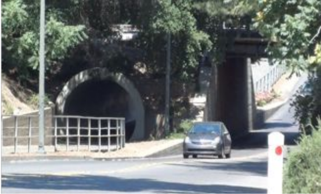
Figure 45. Bicycle Underpass – Davis, California
