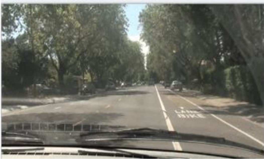
Figure 25. Divided Shoulder for Parking and Bicycling – Palo Alto, California
