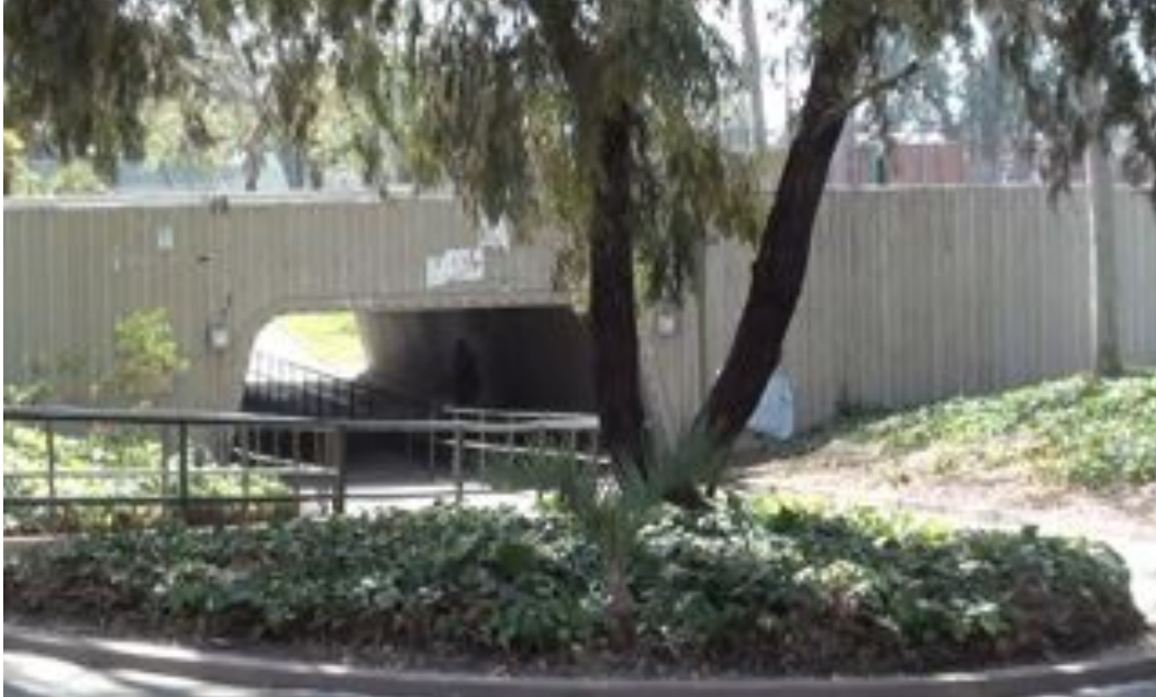
Figure 46. Underpass for Bicycle Path #1 – Santa Barbara, California
