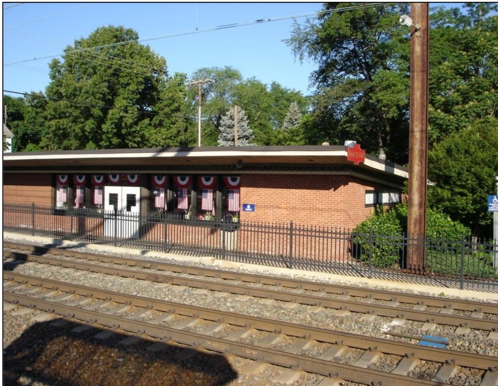
Figure 15: Example of platform edge fencing.
