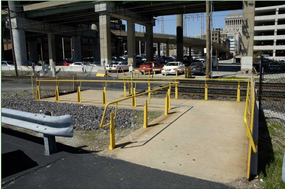
Figure 8: Example of railing used to delineate the desired crossing path for pedestrians.
