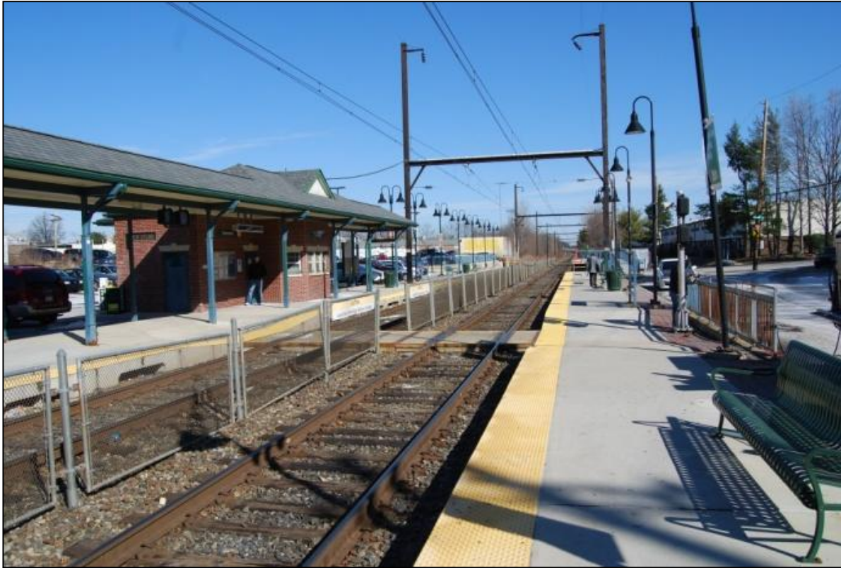
Figure 11: Example of intertrack fencing with crossing surface providing for desired pedestrian movement between passenger platforms.
