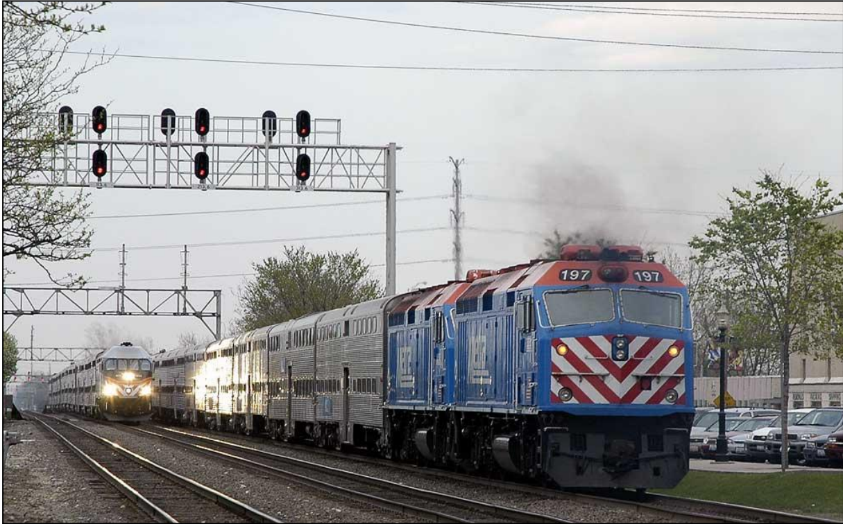
Figure 3: This multi-track railroad features local and limited-stop passenger service.
