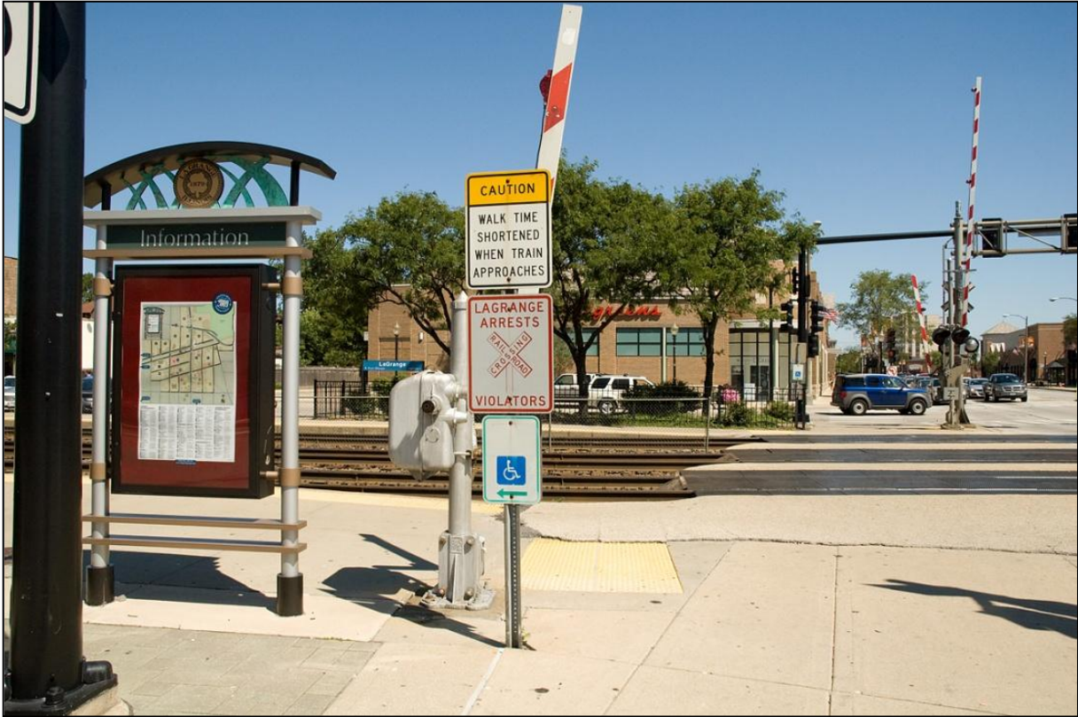
Figure 7: Example of the use of streetscape features, such as the “Information” sign, to enhance the effectiveness of a pedestrian gate by making it more difficult to walk around the warning device.
