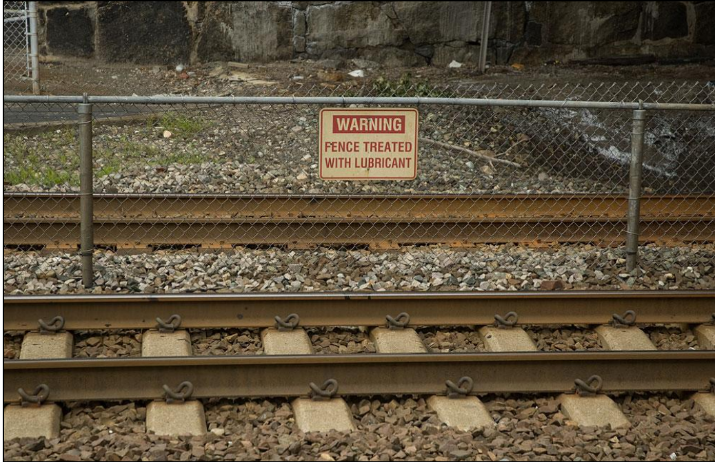
Figure 16: Example of signing and strategy to reduce “fence-jumping” by regular commuters who stubbornly insist on using a favorite shortcut.
