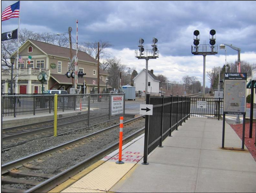
Figure 12: Installation of station signing and channelizing fencing to guide pedestrians away from the station platform and toward the desired safe crossing point at the end of
