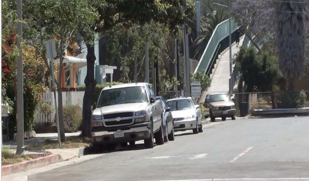
Figure 41. Pedestrian Overpass across US 101 – Santa Barbara, California
