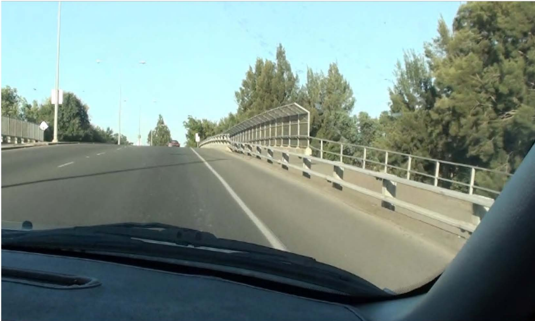
Figure 48. Bicycle Lane on Highway Bridge – Davis, California
