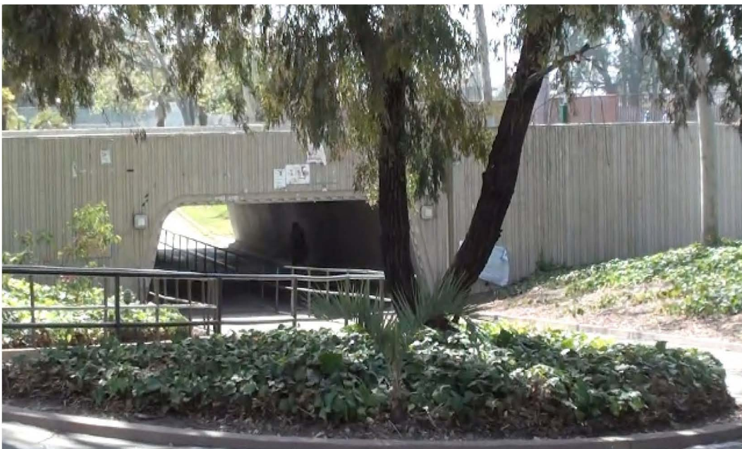
Figure 46. Underpass for Bicycle Path #1 – Santa Barbara, California
