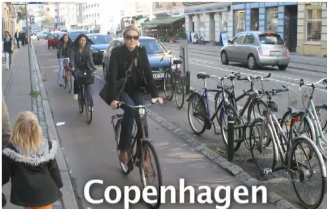
Figure 12. Separate Walking, Bicycling and Auto Facilities – Copenhagen, Denmark
