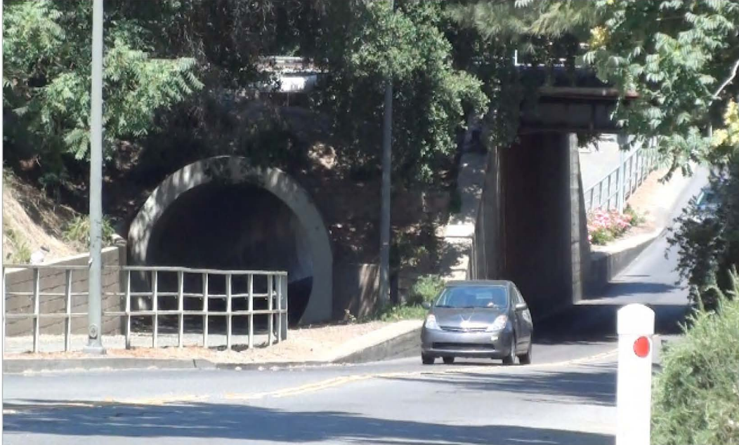
Figure 45. Bicycle Underpass – Davis, California
