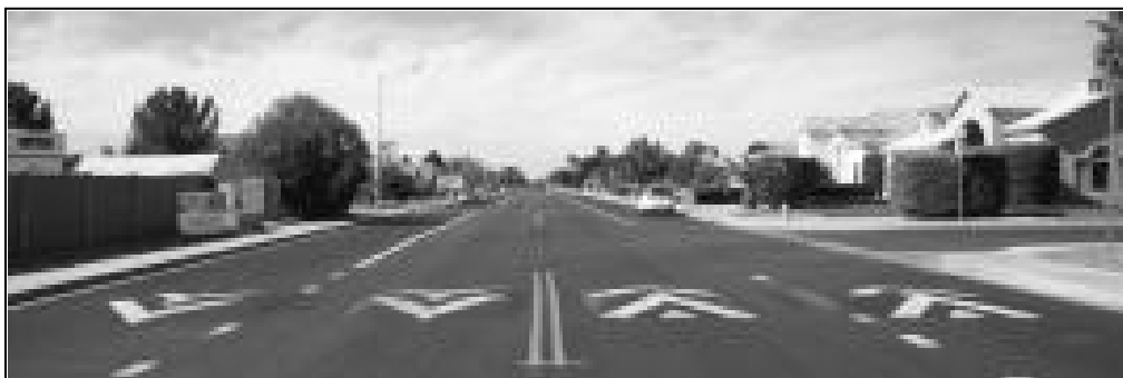
Figure H6 Example of speed cushion layout that could be used at a multi-lane situation
