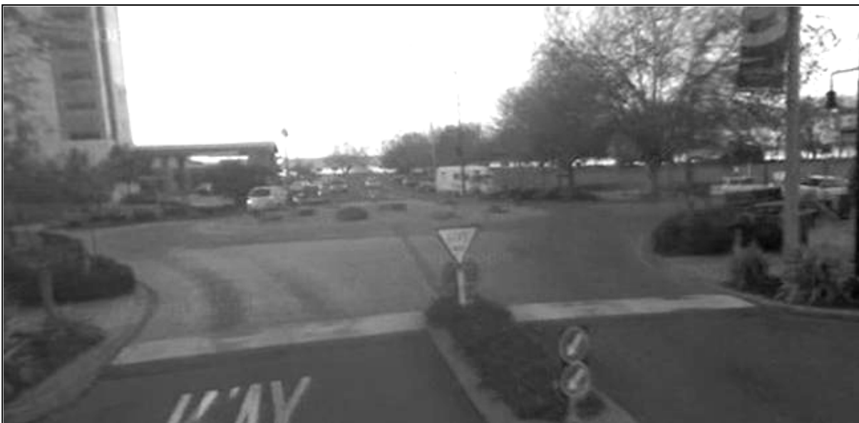
Figure 5.4 Whakahue Street–Tutanekai Street intersection in the Rotorua Central Business District (CBD), where the entire roundabout (single-lane) is constructed as a raised platform, giving a low-speed environment that is conducive to pedestrians
