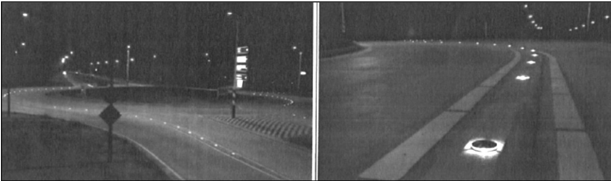
Figure I29 Example of road lighting (LED) to improve visibility of the lane dividers
