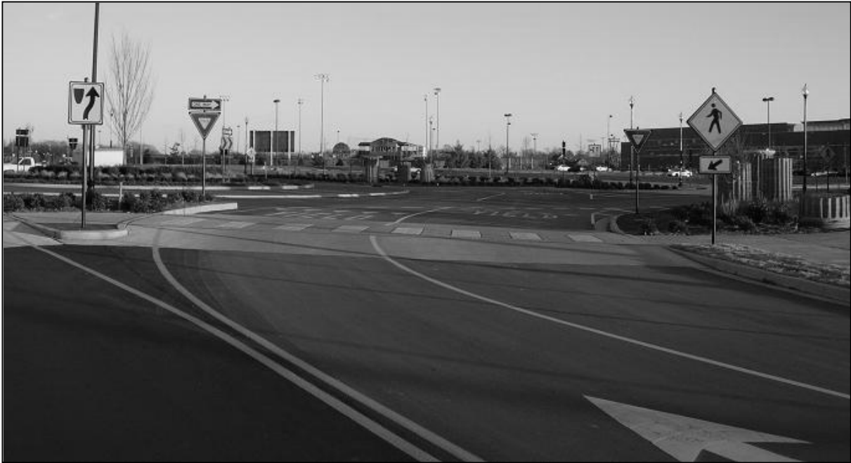
Figure 7.28 A multi-lane zebra crossing on a short raised platform at an unidentified roundabout in the US
