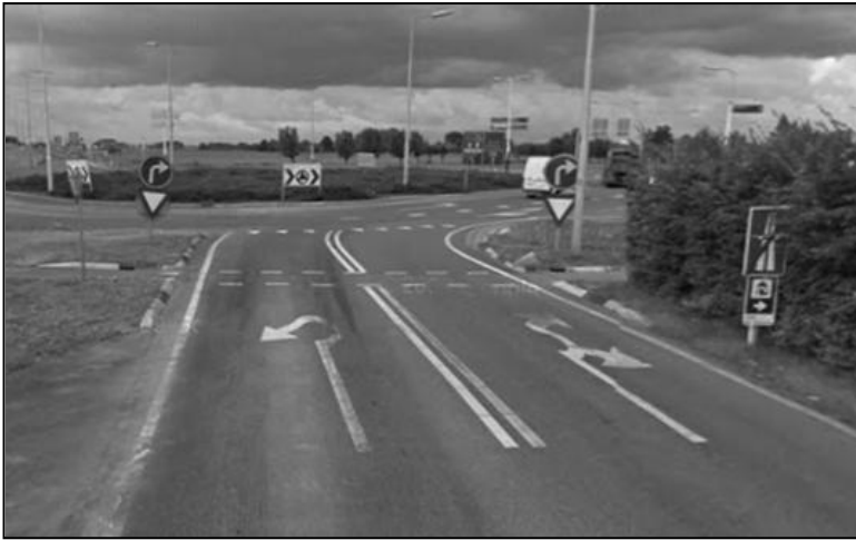
Figure 8.16 Street view of the Rien Cock Ovonde-Provinciale Weg intersection: this five-arm junction is best described as a partial turbo-roundabout, as not every approach has lane dividers – a minor road approach with paint markings only is shown (photo courtesy of Google Maps)
