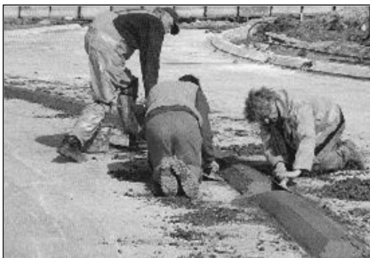
Figure 8.23 In situ construction of the mountable lane dividers: shaping the dividers (CROW 2008)
