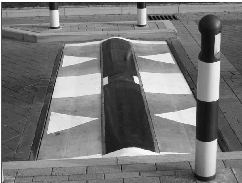
Figure 7.14 Typical example of a Transcalm device (photo supplied by Dunlop Transcalm Ltd)
