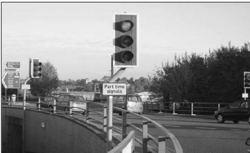
Figure 5.12 Part-time signals in the UK at a motorway junction (DfT 2009)
