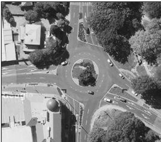
Figure 3.11 Example of a roundabout built with minimal regard for speed control: Riccarton Road and Deans Avenue in Christchurch (photos courtesy of Google Maps)
