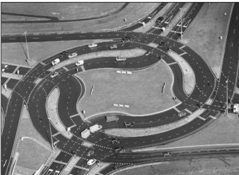
Figure 5.11 Model of a signalised turbo-roundabout (see chapter 8) currently operating in The Netherlands
