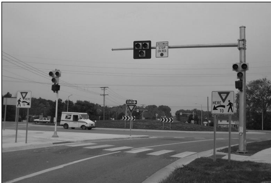
Figure 5.15 A Hawk signal at a two-lane entry to a roundabout in Michigan in the US
