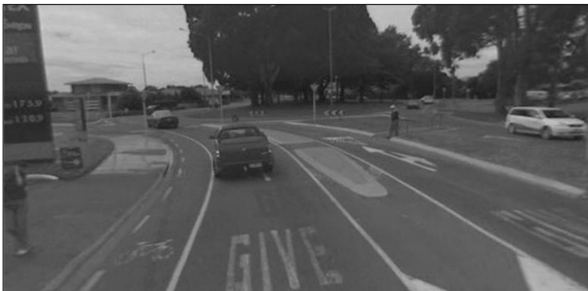
Figure 5.19 Harewood Road eastbound approach to a double-lane roundabout at its intersection with Highsted Road in Christchurch.
