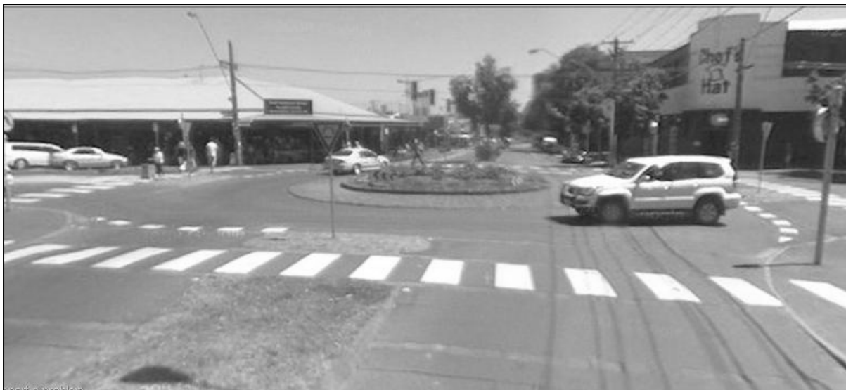
Figure 7.27 The Cecil Street-Coventry Street roundabout in Port Phillip, Melbourne, Australia: conventional raised platforms with zebra crossings on each of the four arms (photo courtesy of Google Maps)
