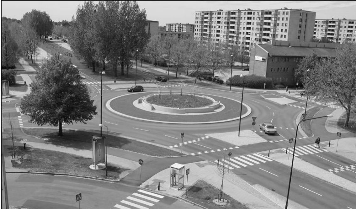
Figure 7.32 The Lorensborgsgatan–Stadiongatan roundabout in Malmö, Sweden (left-hand drive): 100mm high raised platforms are provided on each arm to facilitate the pedestrian and cycle path crossing points around the perimeter of the roundabout (photo provided by Transport Department, City of Malmö)
