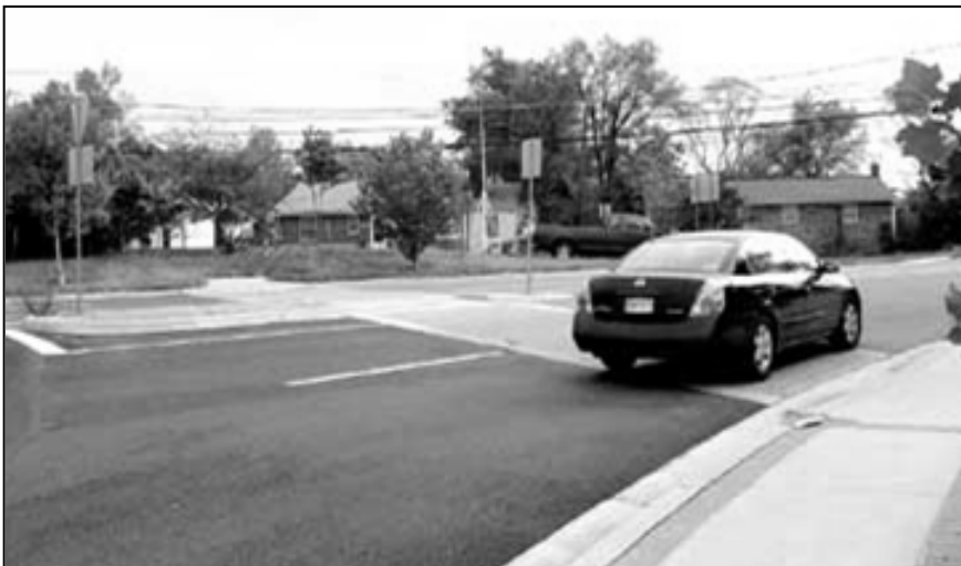
Figure 7.1 A low raised speed platform on a two-lane roundabout exit in the US
