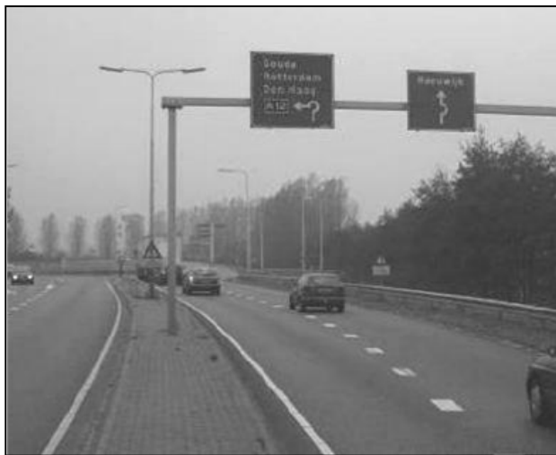
Figure 8.35 Optional overhead signage to be installed 100m in advance of the turbo-roundabout (CROW 2008)
