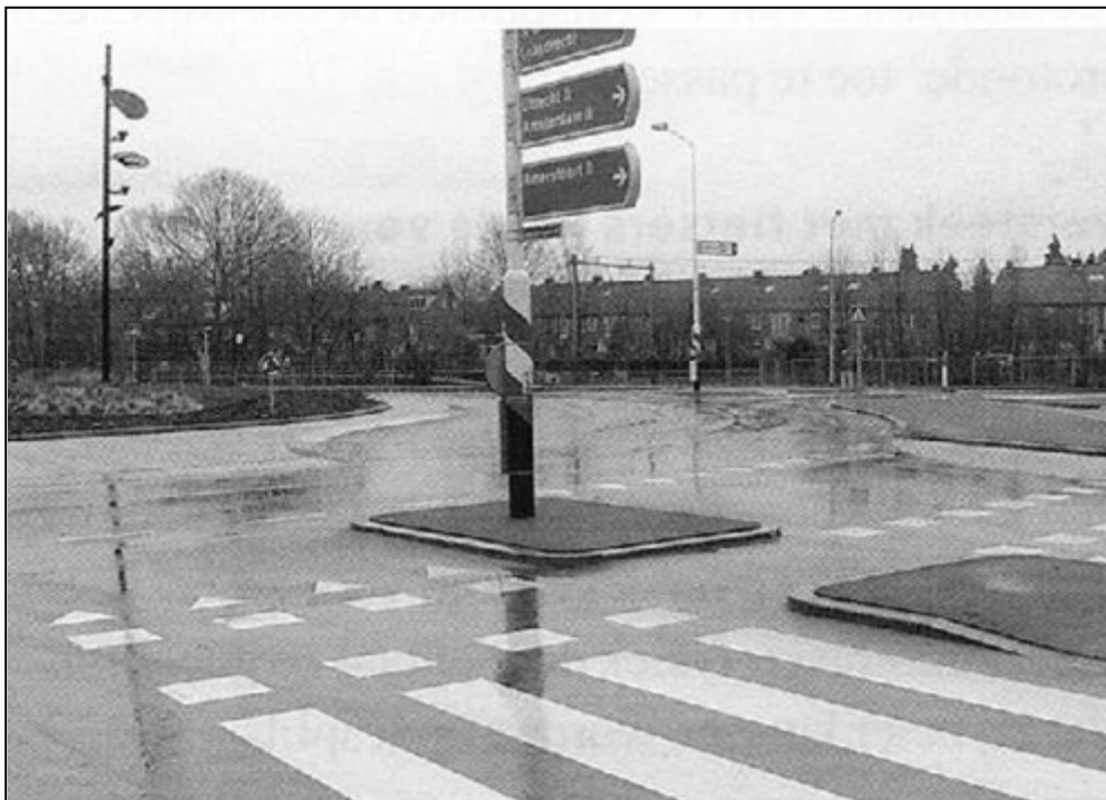
Figure 8.31 Closer view of the markings of the at-grade perimeter paths for cyclists and pedestrians at a Dutch turbo-roundabout - note the small white triangle markings that denote who has priority of way in The Netherlands (CROW 2008)
