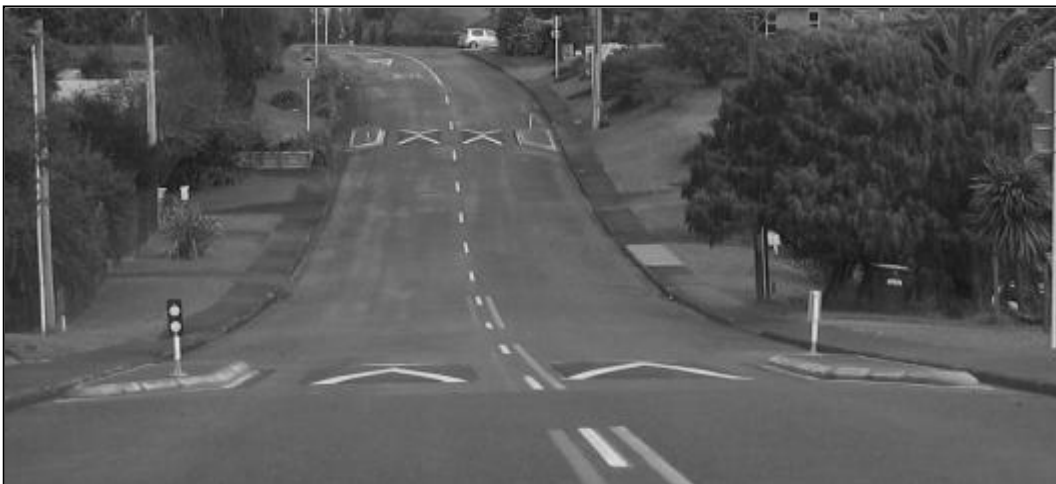
Figure H4 Photo of a speed cushion scheme installed in Waitakere City, Auckland
