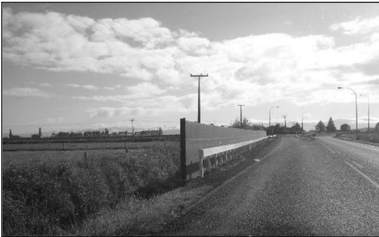
Figure 4.4 The minor road eastbound approach showing the hessian screen at the Paeroa-Tahuna Road-State Highway 27 intersection (photo taken in 2008)
