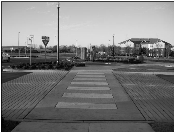
Figure 7.29 Another view of the multi-lane roundabout shown in figure 7.28
