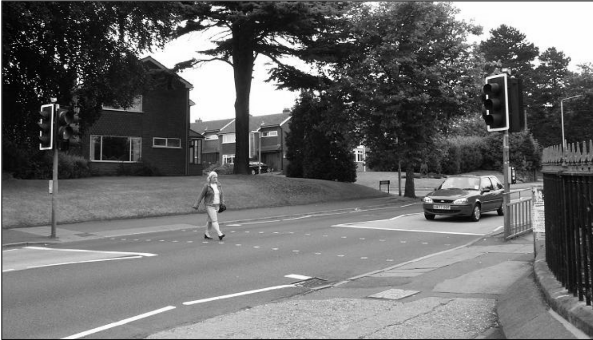
Figure 5.13 A British Pelican crossing, which is a full-time signal arrangement using three-aspect displays facing drivers. This particular example is fitted with nearside displays for pedestrians similar to those used by Puffin crossings (photo from Dudley Metropolitan Borough Council)
