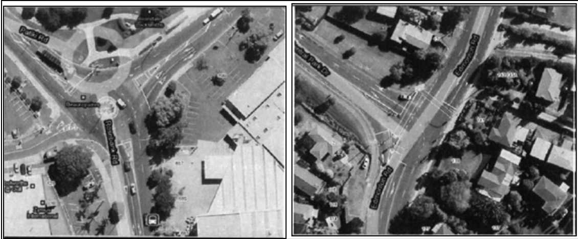
Figure A20 Matched pair 18: Swanson Road-Metcalf Road roundabout (left) and Campbell Road-Wheturangi Road traffic signals (photos courtesy of Google Maps)
