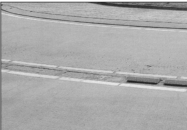
Figure 8.26 Photo of the damage that can occur if lane dividers are glued onto the roadway instead of cast in situ (CROW 2008)
