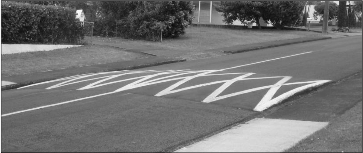
Figure H3 Photo of a MWP speed hump, as commonly installed in some New Zealand jurisdictions
