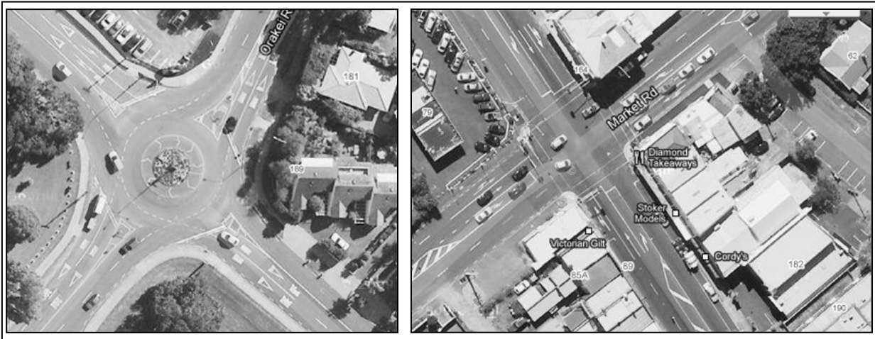
Figure A10 Matched pair 8: Shore Road–Orakei Road roundabout (left) and Great South Road–Market Road traffic signals (photos courtesy of Google Maps)
