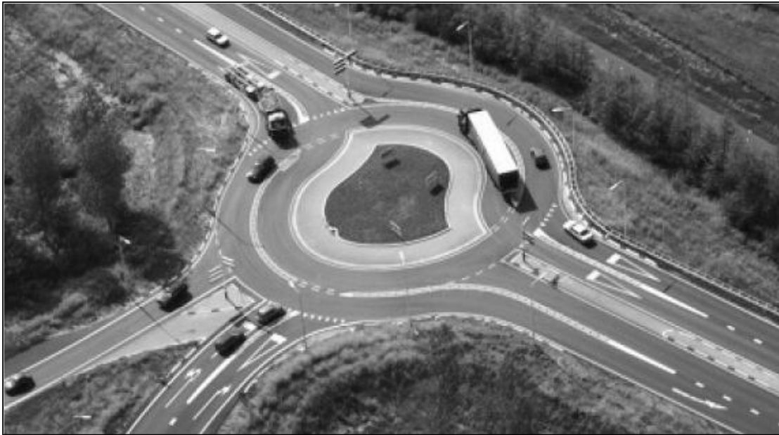
Figure 8.1 A turbo-roundabout in The Netherlands, showing the typical layout (CROW 2008)
