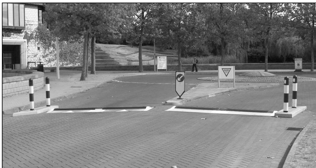
Figure 7.15 Example of a Transcalm in the UK installed near a single-lane roundabout on a busy bus route (photo supplied by Dunlop Transcalm Ltd)
