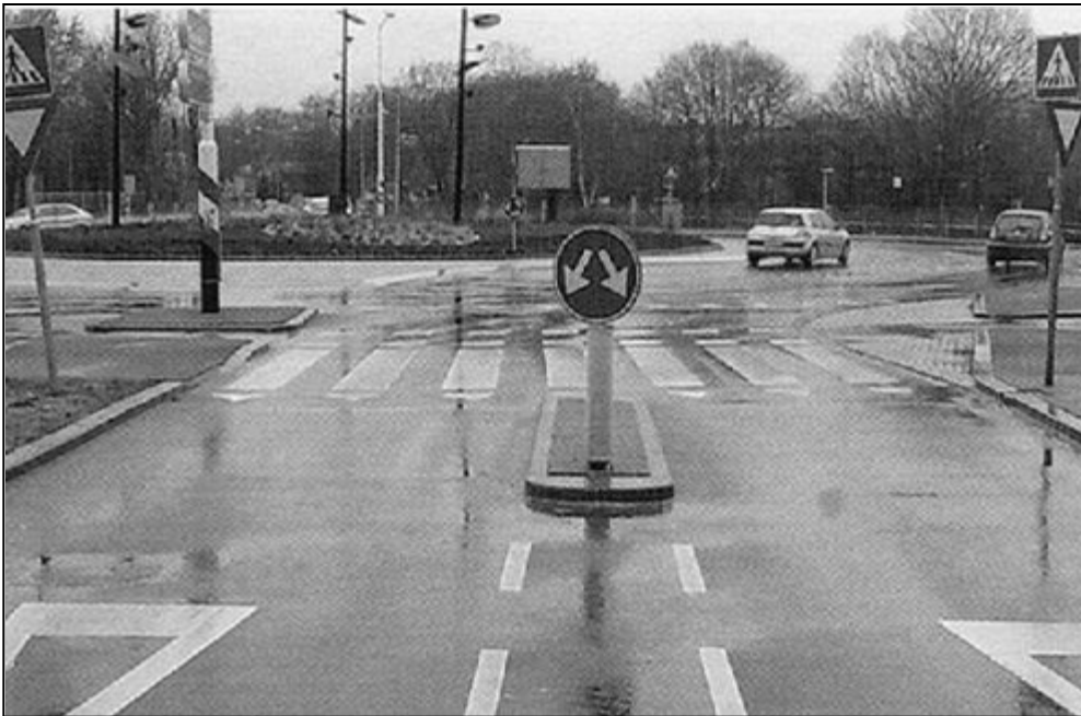
Figure 8.30 Example of a turbo-roundabout with at-grade perimeter paths for cyclists and pedestrians, who have priority over vehicles, much like zebra crossings for pedestrians in New Zealand (CROW 2008)
