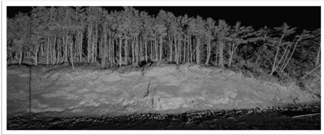
Figure 1.1: 3D laser scan survey point cloud of the Johnson Creek landslide (June 2011).
