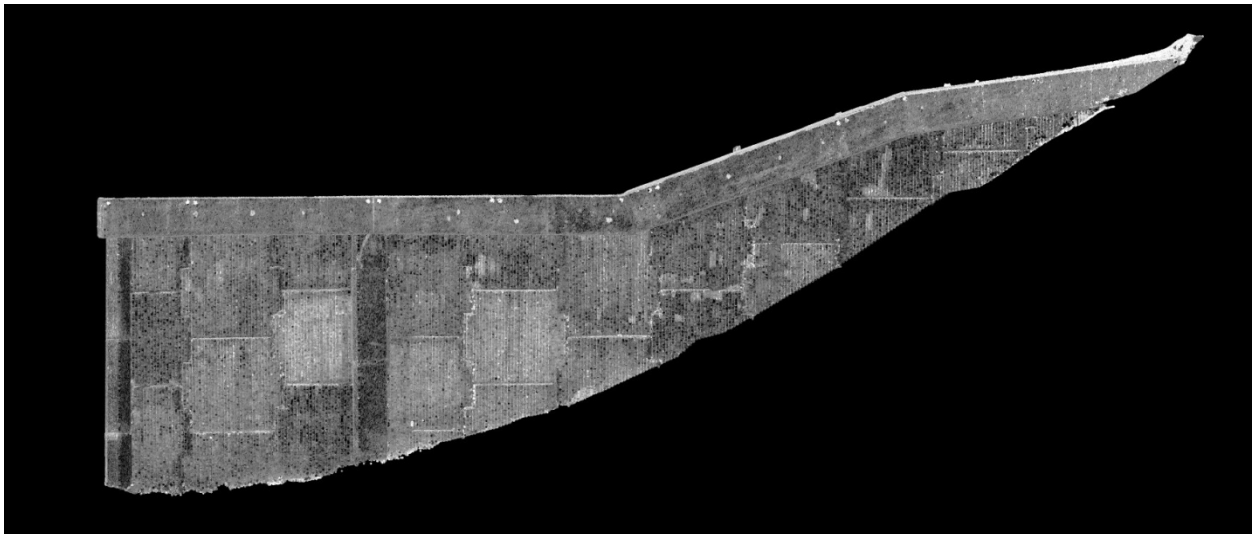
Figure 3.14: Intensity map of MSE wall face between January and February 2011 surveys. Note that the new concrete patches reflect light differently than the worn concrete.
