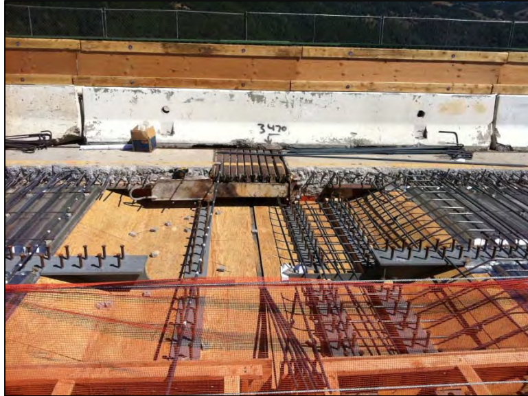
Figure 5.12 Bridge Expansion Bearing Replacement During Deck Widening
