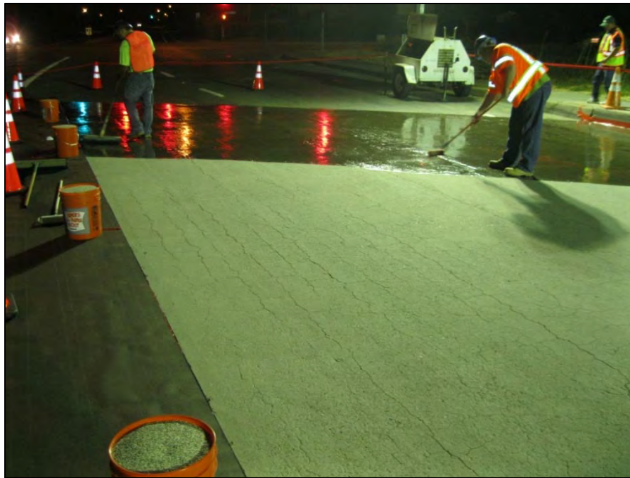
Figure 5.4 Bridge Deck Rehabilitation With Methacrylate Resin Treatment
