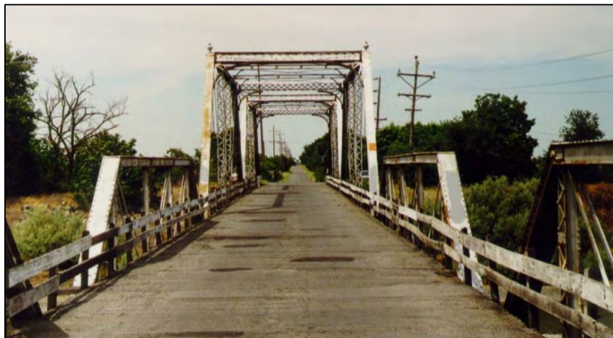
Figure 5.5 Structurally Deficient – Low Deck & Superstructure Condition Rating
