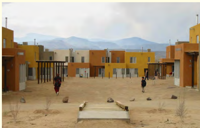
The buildings in Tsigo Bugeh Village are clustered around two plazas, and contain affordable townhouses, a meeting space, a playground, a computer room, a fitness room, and business center. Photo courtesy of the San Juan Pueblo Office of the Governor.
