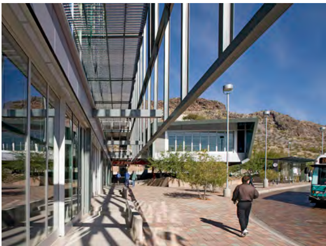
The Tempe, Arizona Transportation Center combines the downtown light-rail stop, the main city bus station, and the state's first "bike station," which offers secure on-site storage and repairs, into one facility. Photo courtesy of City of Tempe and Architekton + Otak.
