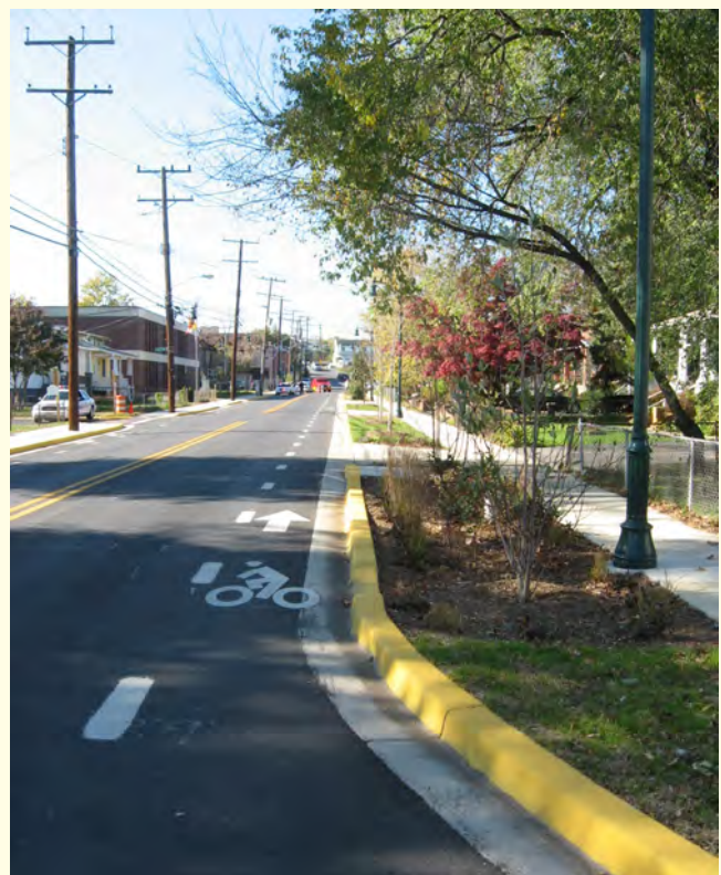
Decatur Street's bike lanes are constructed with permeable materials that allow water to filter through instead of collecting on top. Photo courtesy of Faith Cole.
